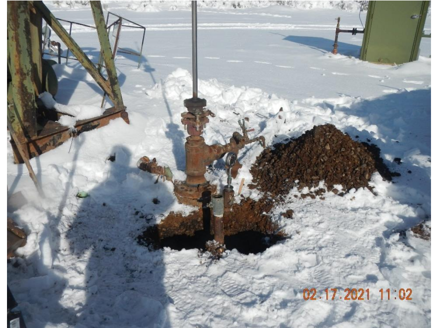
Impacted material observed in excavation around well head.
