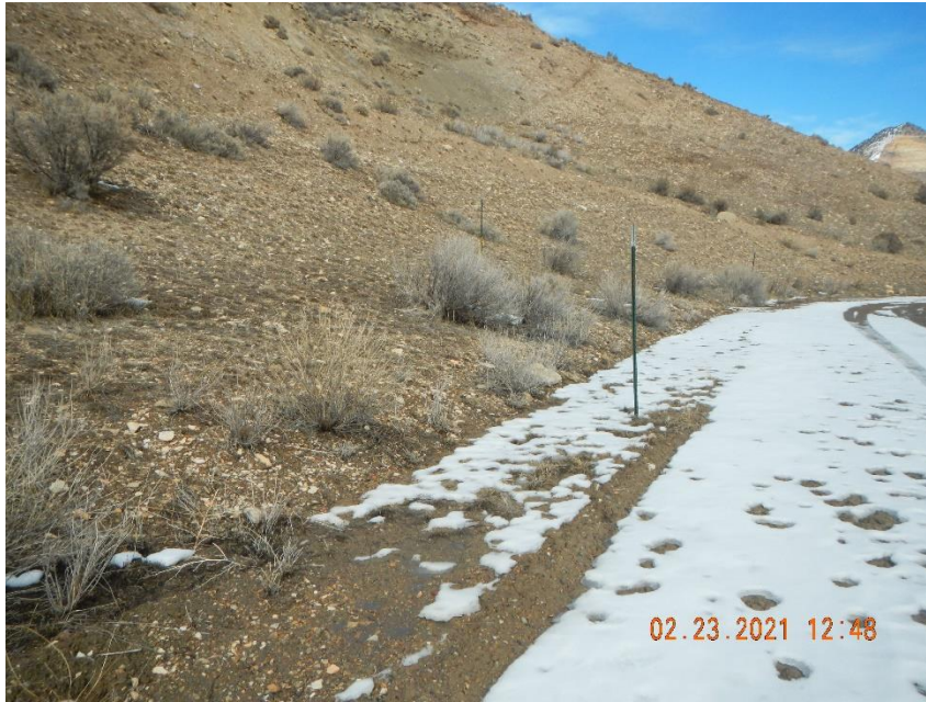
Sediment build up in perimeter ditch.
