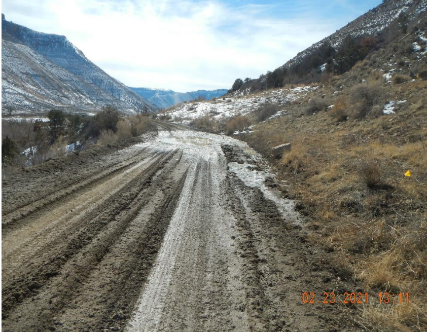
N39.55096 W108.12064 Rut damage in ditch. Water not draining off road into culvert or ditch.
