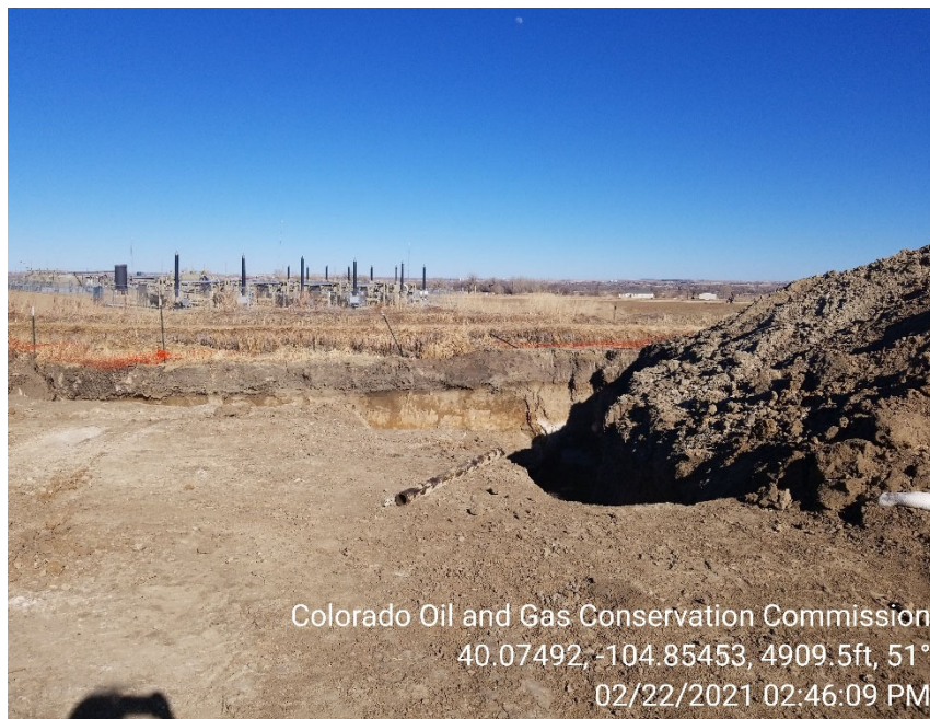
Photo 1 – Spill area. No fencing around open excavation
