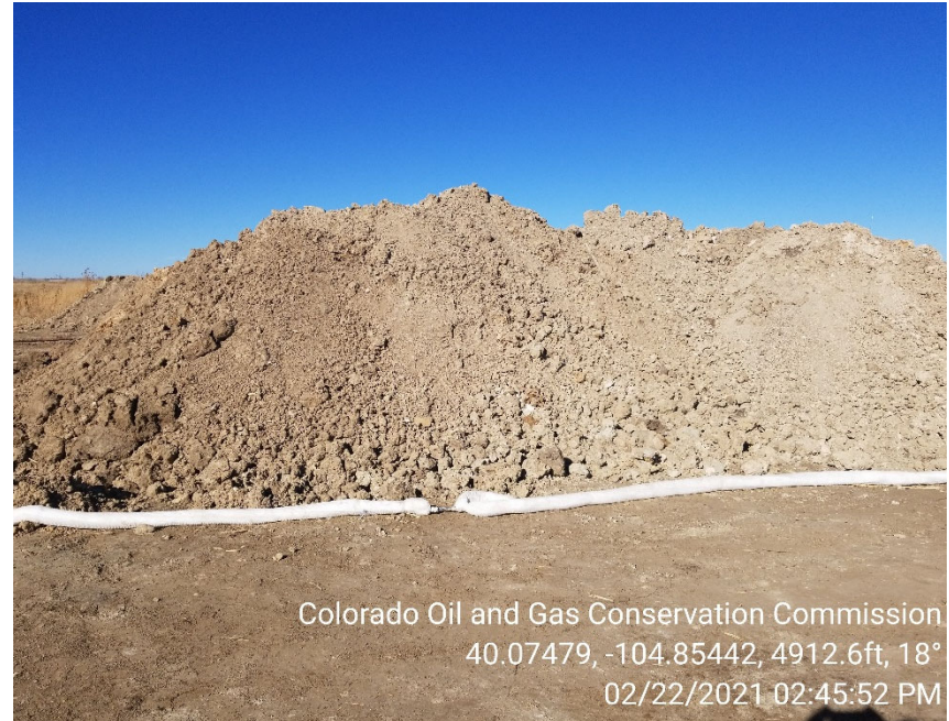
Photo 6 – Soils stored on location; BMPs inadequate to contain runoff
