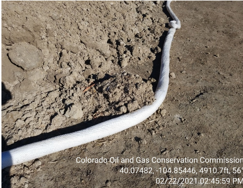
Photo 5 – Soils stored on location; BMPs inadequate to contain runoff
