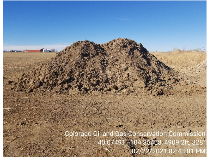
Photo 4 – Soils stored on location; BMPs inadequate to contain runoff
