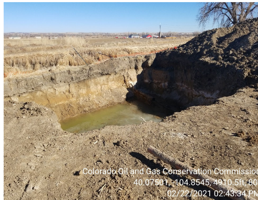
Photo 2 – Spill area; groundwater observed in the excavation
