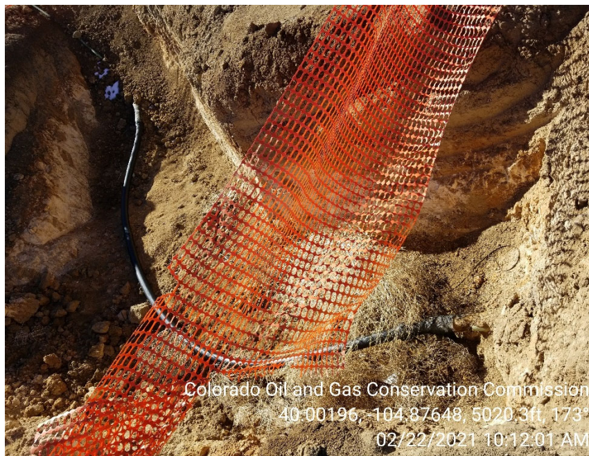
Photo 5 – Repaired flowline in open excavation
