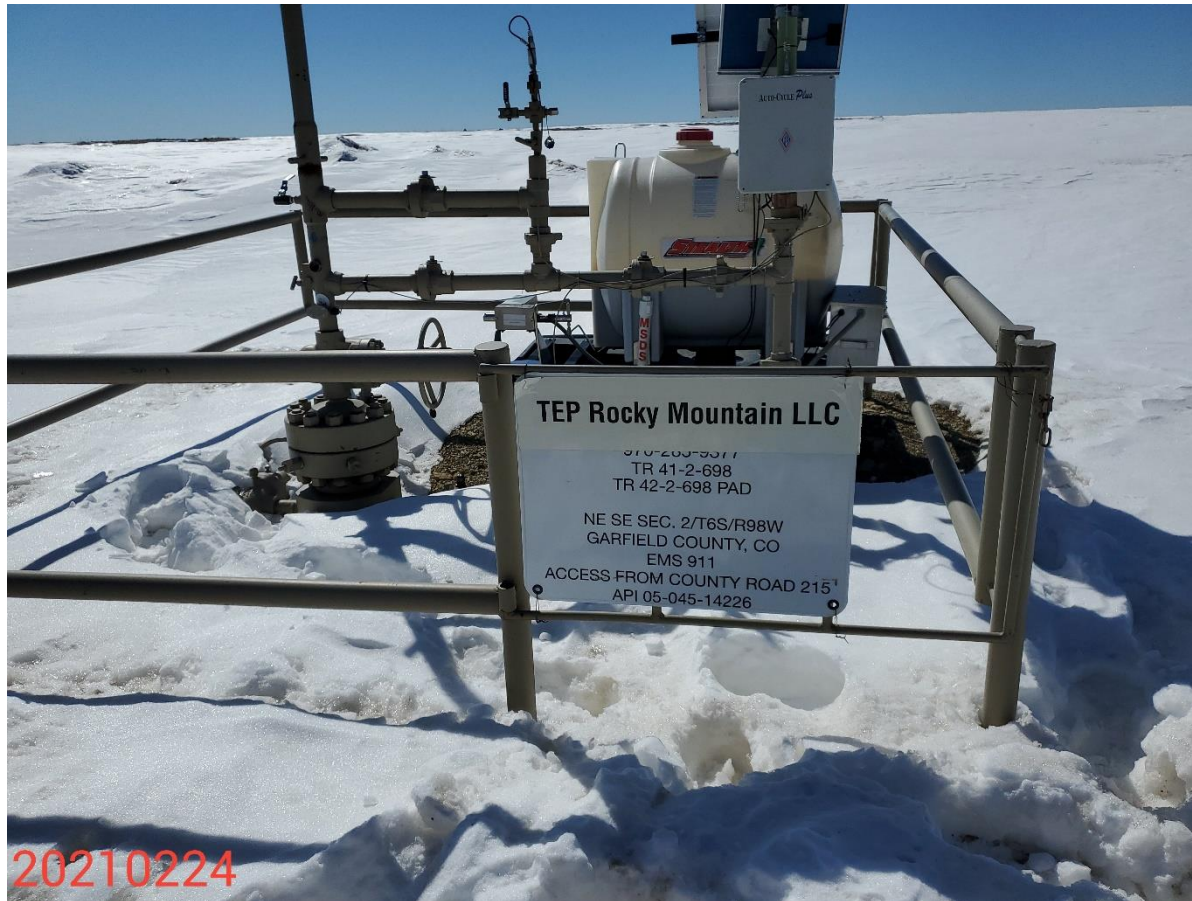
Photo 1: Photo shows well head. Emergency contact number partially covered by sticker.
