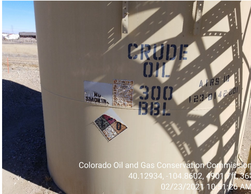
Photo 3 – NFPA label peeling from crude oil tank and no longer legible.
