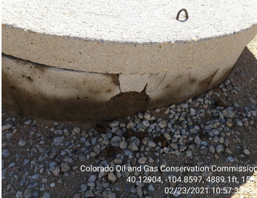
Photo 9 – Cracks/staining visible on produced water vault.
