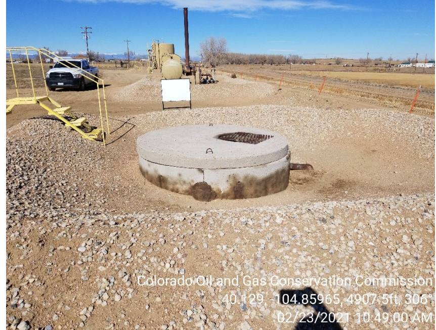
Photo 10 – Cracks/staining visible on produced water vault.
