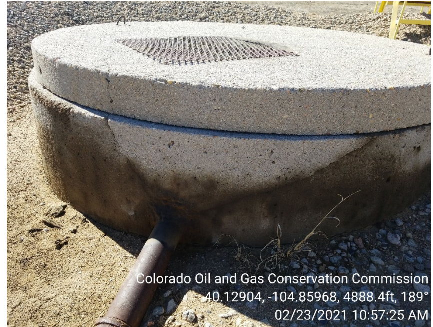
Photo 8 – Cracks/staining visible on produced water vault.
