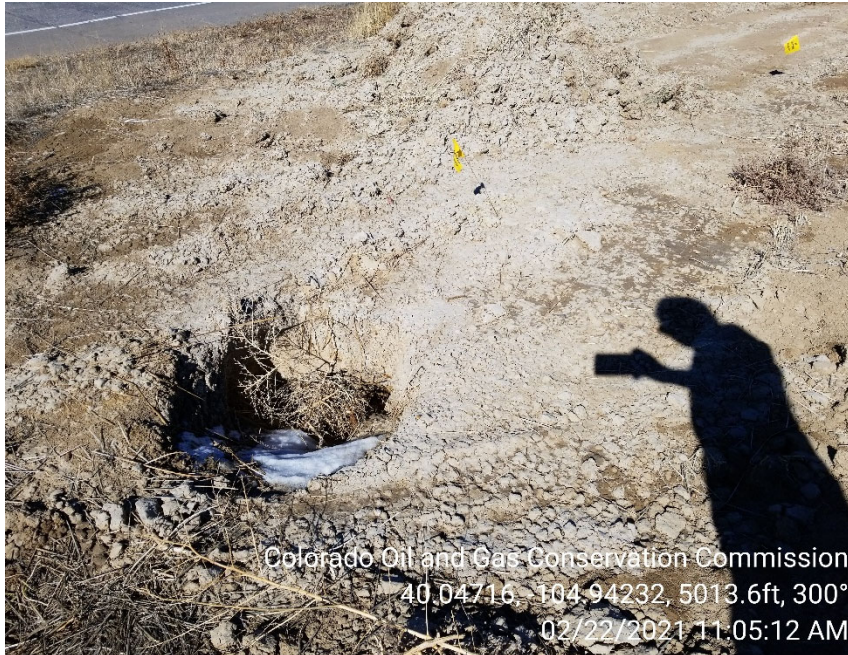
Photo 1 – Potholed spill area
