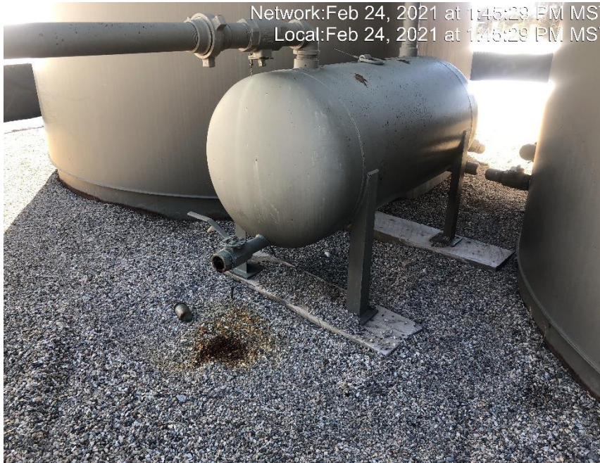
Photo #2968 Stained soils under ECD fluid knock out drain valve.
