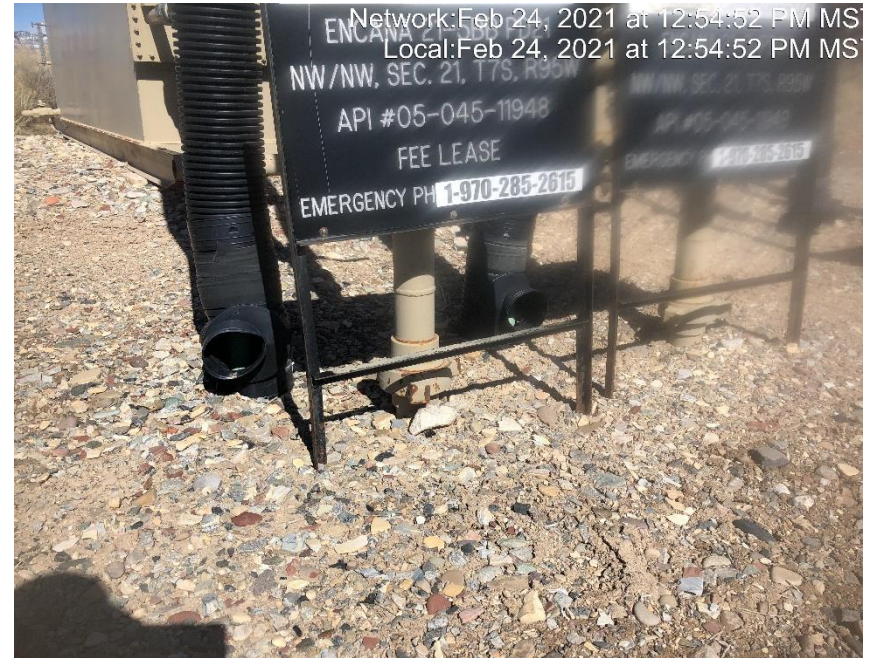
Photo #2961 Flow line heating insulation open ended and not capped.
