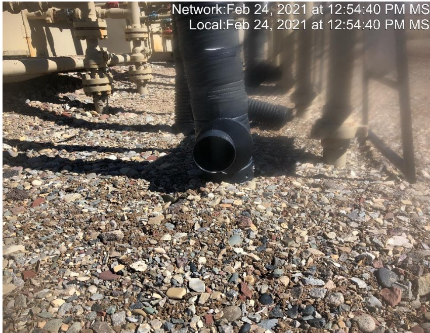
Photo #2960 Flow line heating insulation open ended and not capped.
