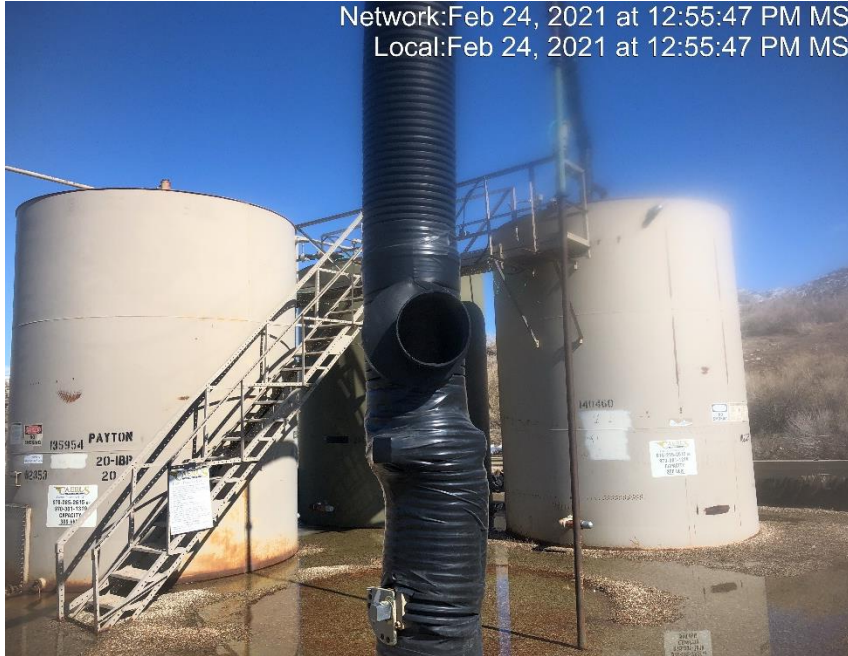
Photo #2962 Flow line heating insulation open ended and not capped.
