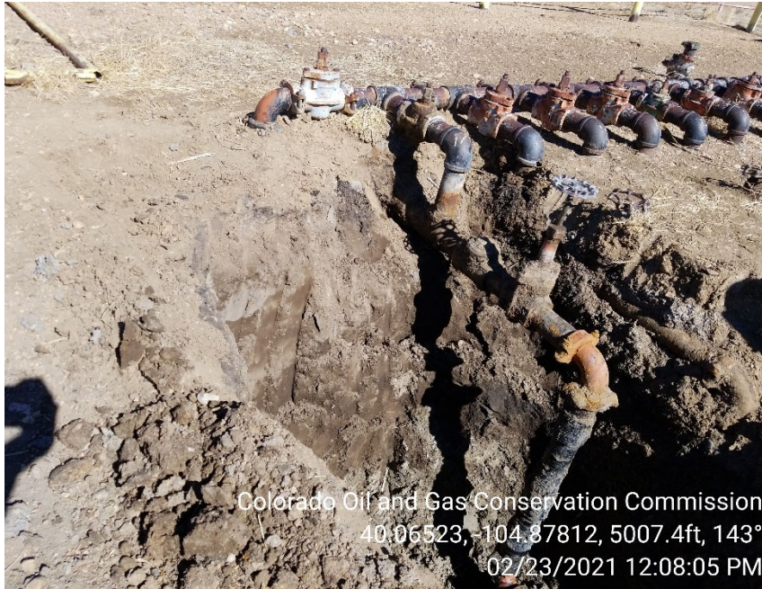
Photo 1 – Spill excavation with exposed flowline. Impacts still visible insitu.
