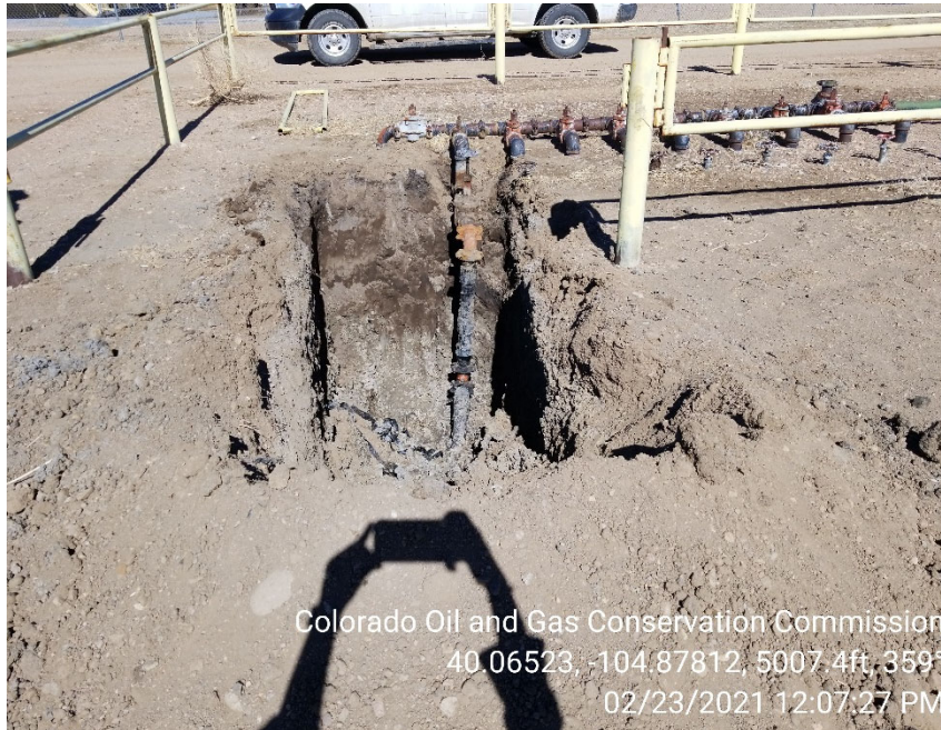
Photo 3 – Spill excavation with exposed flowline. Impacts still visible insitu.
