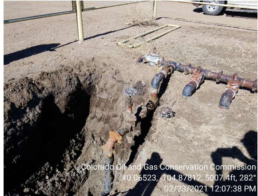
Photo 2 – Spill excavation with exposed flowline. Impacts still visible insitu.
