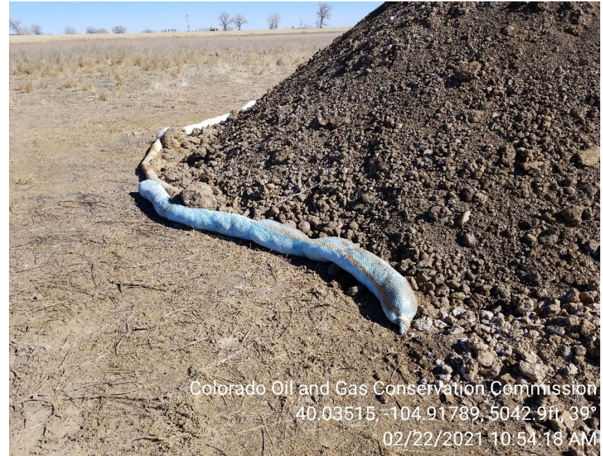
Photo 6 –BMPs inadequate to prevent contamination of stormwater, surface water, Groundwater, and soil
