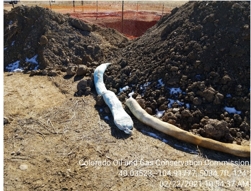
Photo 8 – BMPs inadequate to prevent contamination of stormwater, surface water, Groundwater, and soil
