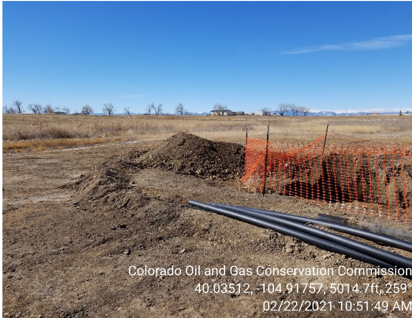
Photo 1 – Spill excavation area. Fencing present around open excavation.
