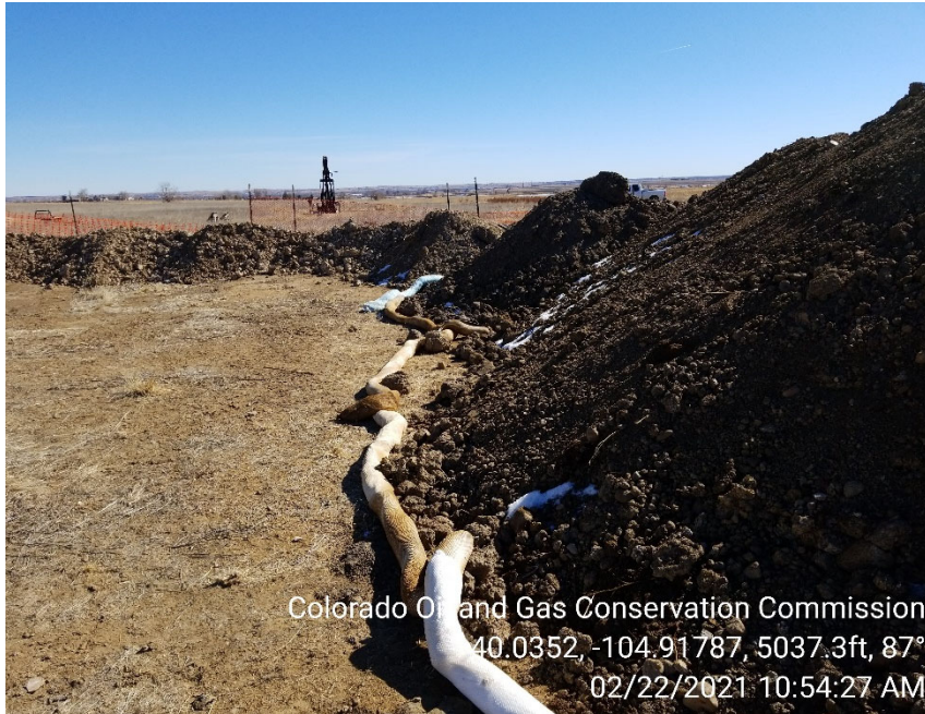
Photo 7 – BMPs inadequate to prevent contamination of stormwater, surface water, Groundwater, and soil
