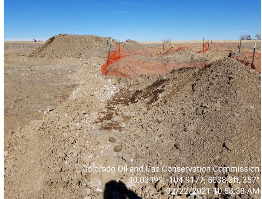
Photo 2 – Spill excavation area. Fencing present around open excavation. Soils stored on site.
