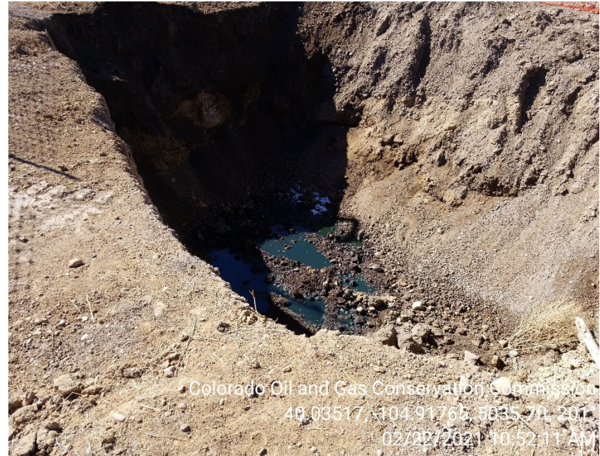
Photo 4 – Free product present in open excavation.
