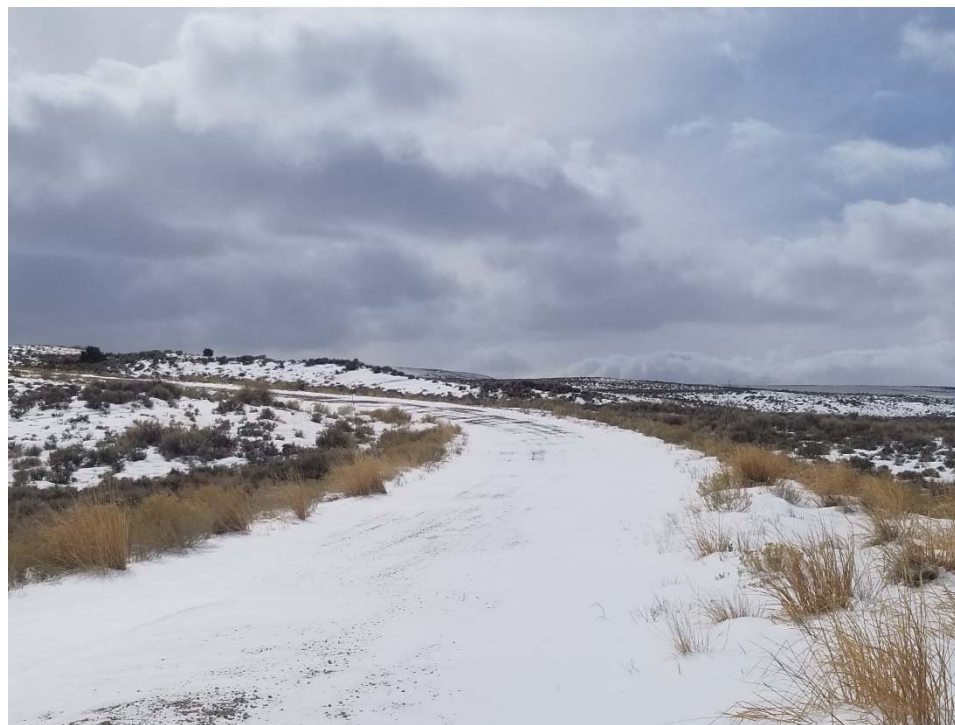
Photo 1. Roads not maintained for winter.
