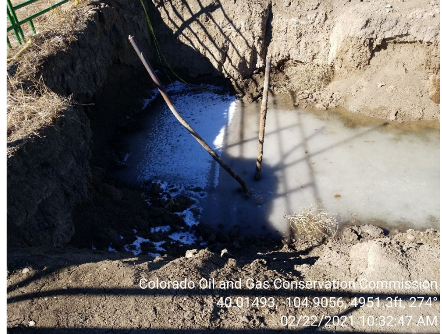
Photo 2 – Spill excavation area. Flowline debris present in excavation.
