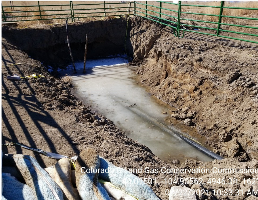
Photo 1 – Spill excavation area. Fencing surrounding open excavation. Groundwater observed in excavation.
