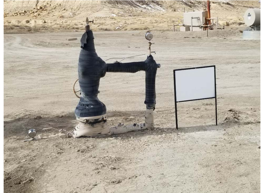
Photo 2. No bradenhead access apparent.
