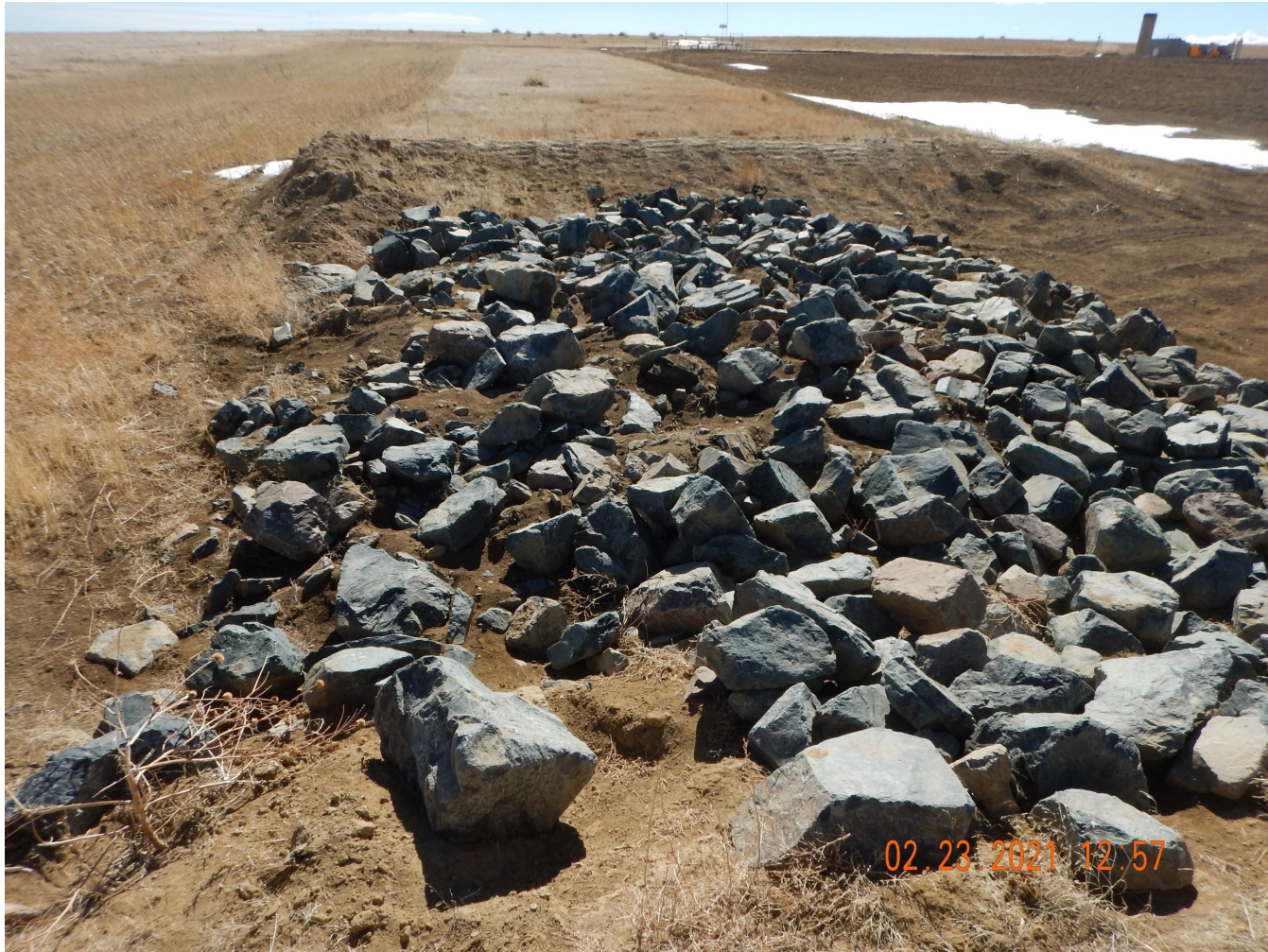
Photo 6. Photo taken from the northeastern location, facing South. Photo illustrates the stabilized outlet, which appears to be in need of maintenance with the accumulation of sediment within the rip-rap material.
