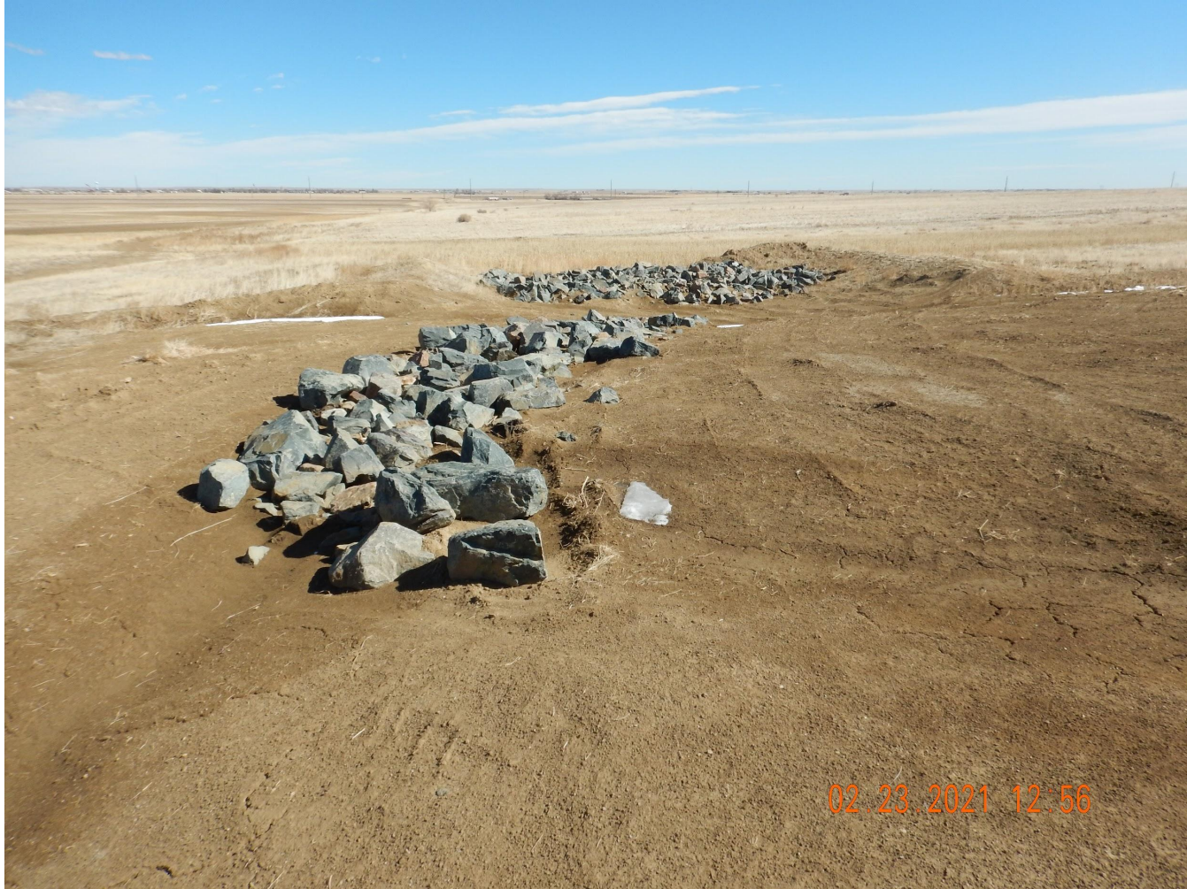
Photo 5. Photo taken from the northeastern location, facing East. Photo illustrates rip-rap functioning as a check dams, which is directed to a stabilized outlet.
