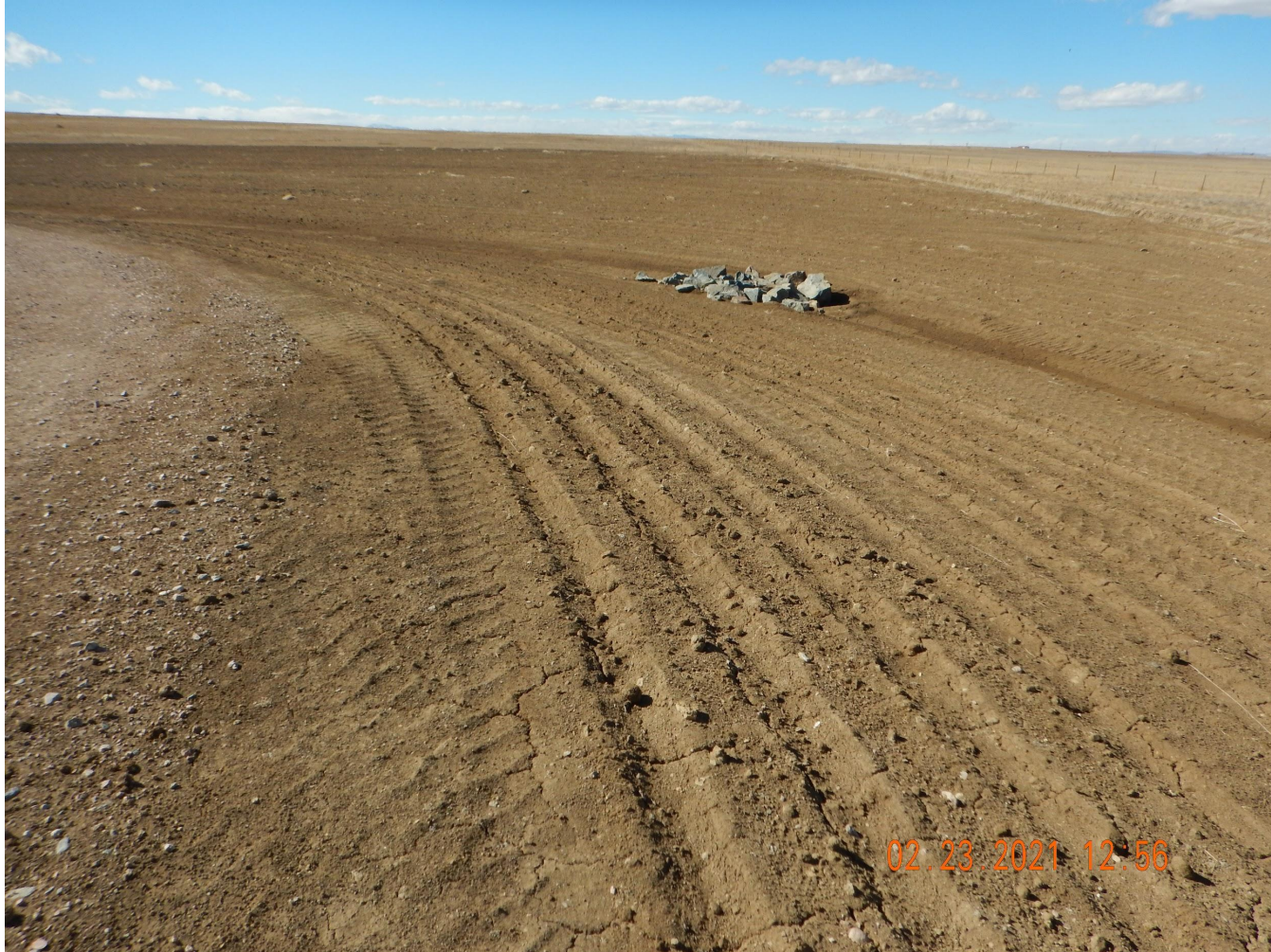
Photo 4. Photo taken from the northern location, facing West. See comment under Photo 1. Photo illustrates rip-rap functioning as a check dam.
