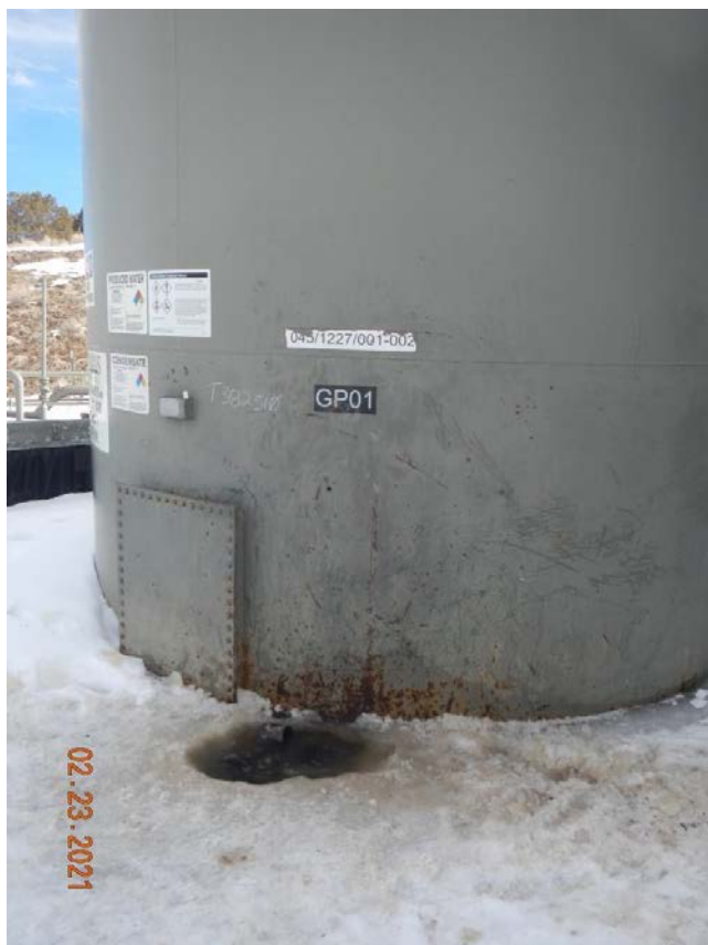
Photo#2: Valve may be leaking.
