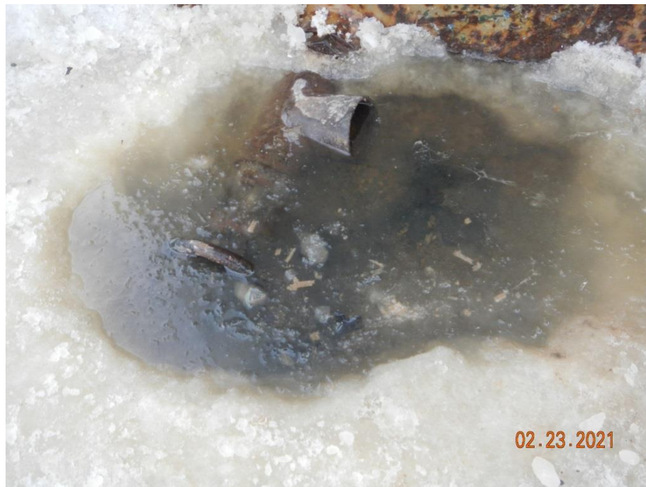
Photo#3: Valve may be leaking.
