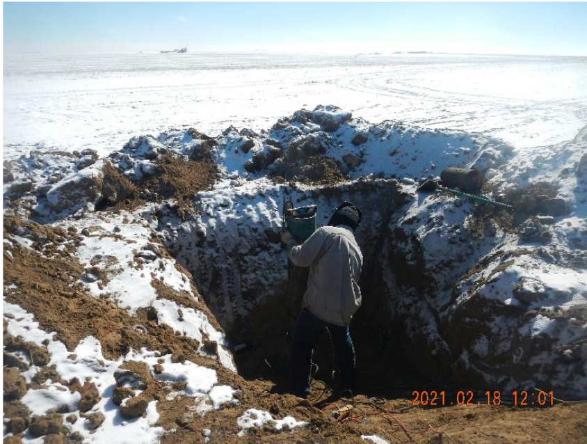
Photo 7: Welding extension into place.
