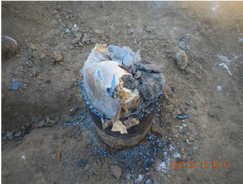
Photo 3: Cut off surface casing to solid pipe and exposed cement plug.
