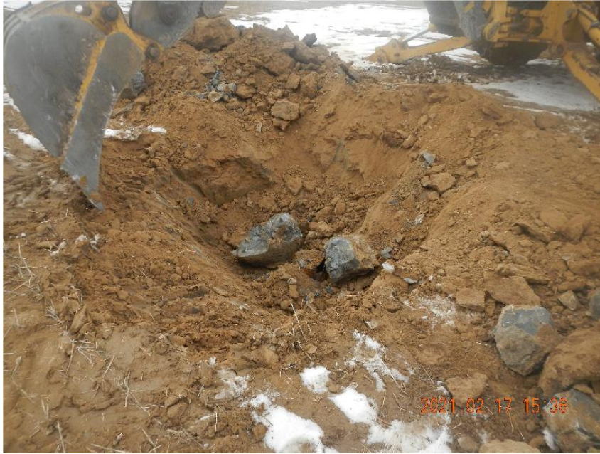
Photo 1: Excavating previously cut and capped surface casing.
