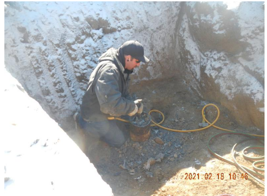
Photo 4: Removing cement plug in surface casing.
