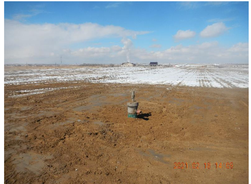
Photo 10: Wellhead completed and ready for rig move in.
