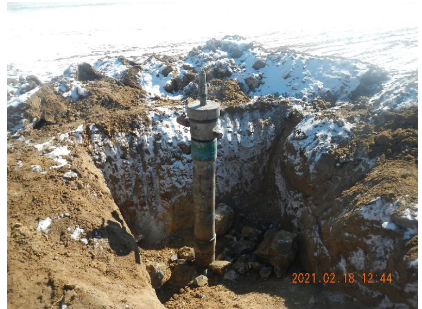
Photo 8: Installed wellhead on surface casing extended to surface.
