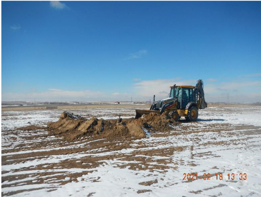
Photo 9: Backfilling excavate area.
