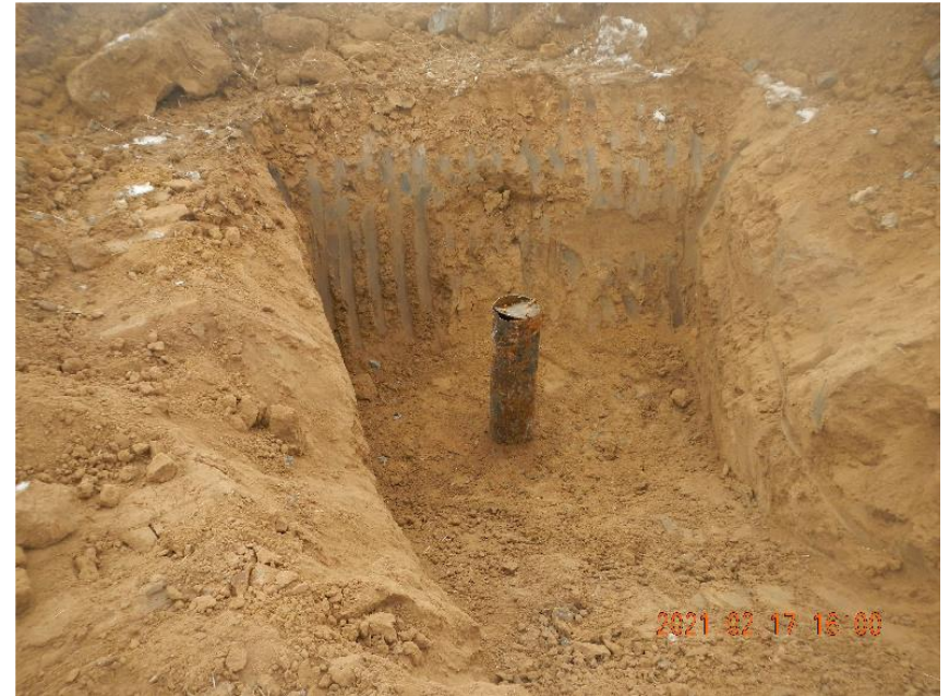
Photo 2: Surface casing and cap.
