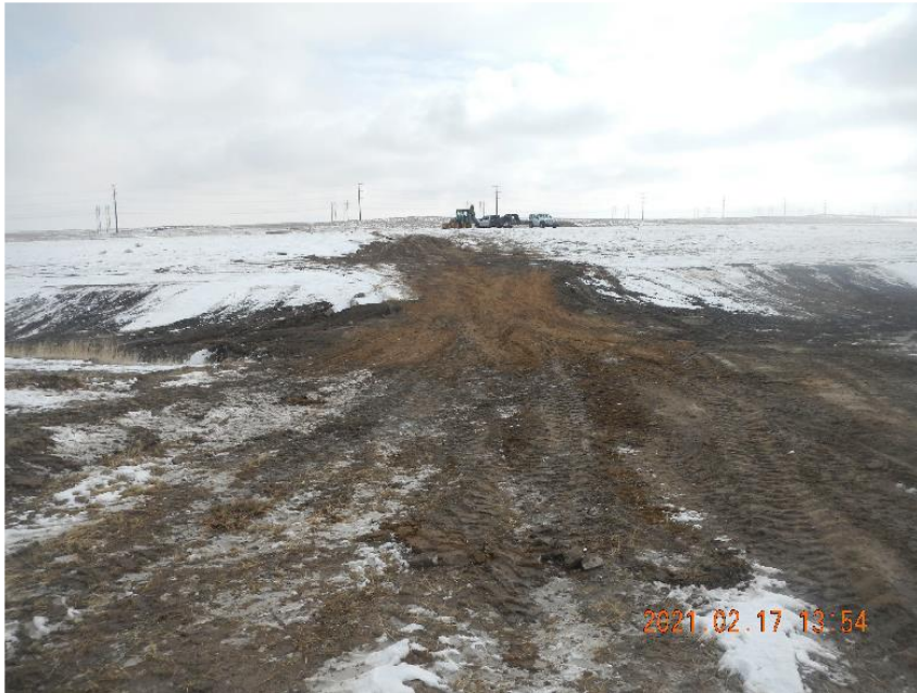
Photo 9: Top view of repaired access road.
