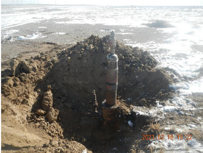
Photo 3: Braden Head plumbed to surface.
