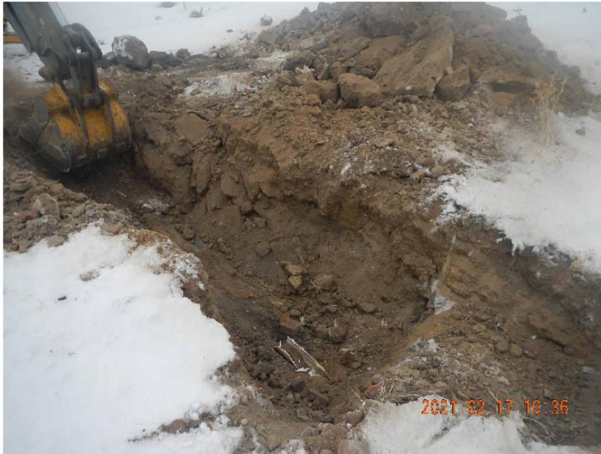
Photo 5: Trench access road for culvert to repair wash out.
