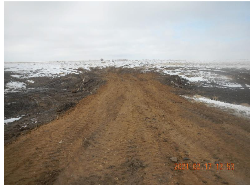
Photo 8: Spreading road base over repair to stabilize area.
