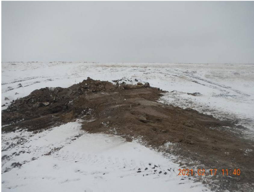
Photo 7: Backfilling and compacting fill over culvert.
