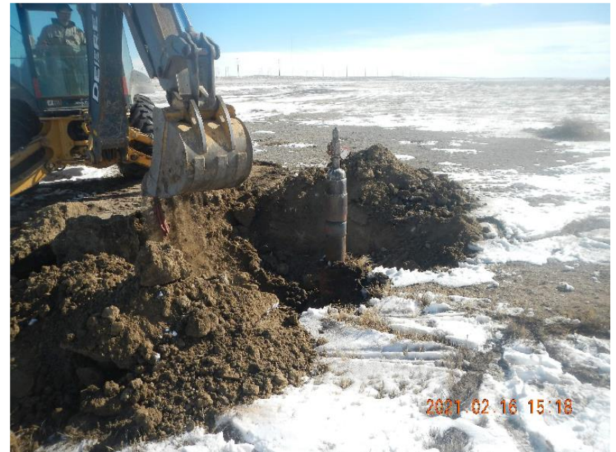
Photo 2: Excavating around wellhead to plumb in Braden Head to surface.
