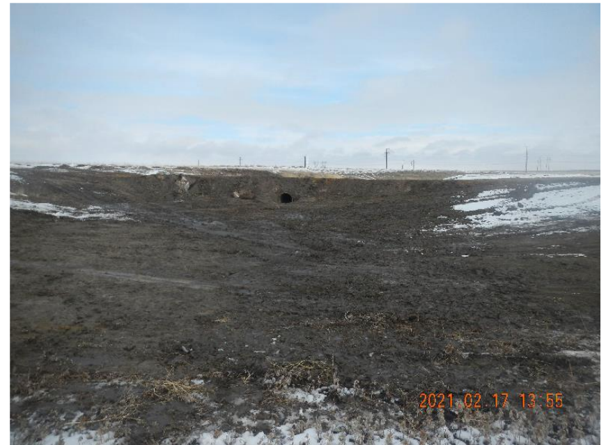
Photo 10: Lower view of repaired road with new culvert.
