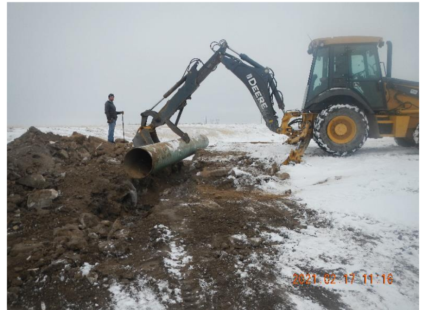
Photo 6: Laying in new culvert.
