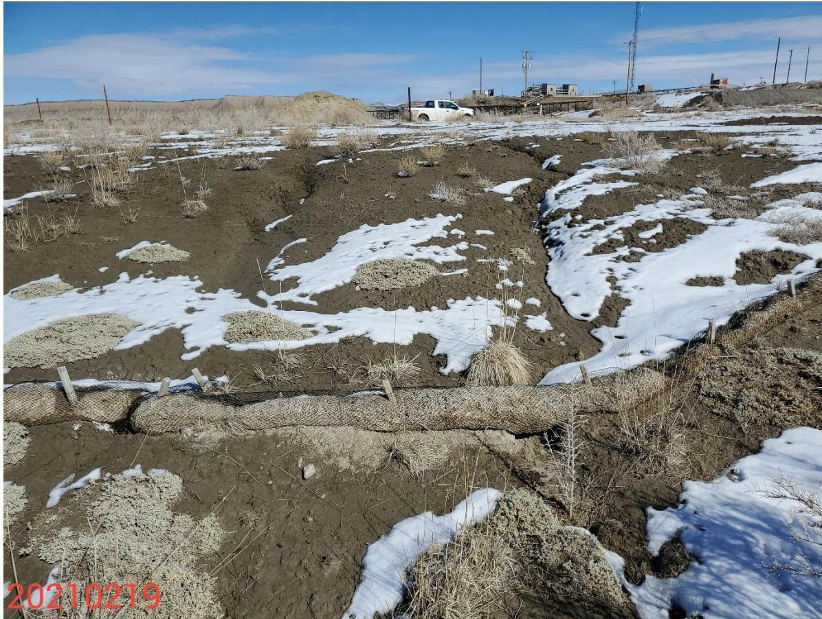
Photo 6: Photo taken from the southern areas of the Location, facing north. Photo shows stormwater and erosion control measures are missing or insufficient to stabilize soils.
