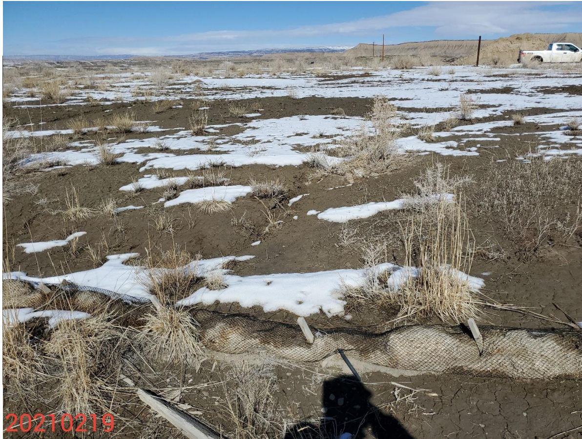
Photo 8: Photo taken from the southern areas of the Location, facing north. Photo shows stormwater and erosion control measures are missing or insufficient to stabilize soils.
