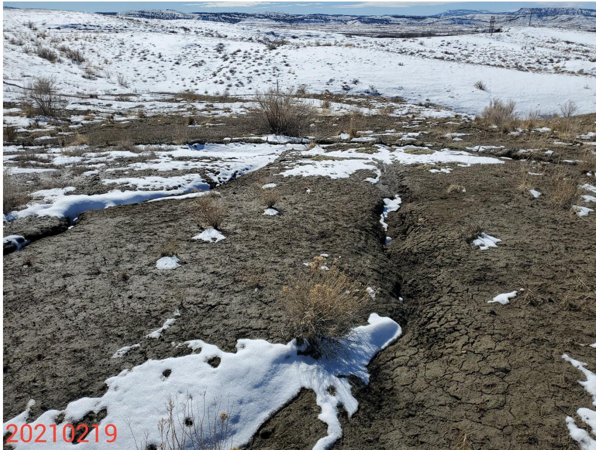
Photo 3: Photo taken from the southern areas of the Location, facing south. Photo shows areas of the Location where vegetative establishment is not occurring, and stormwater and erosion control measures are missing or insufficient to stabilize soils.
