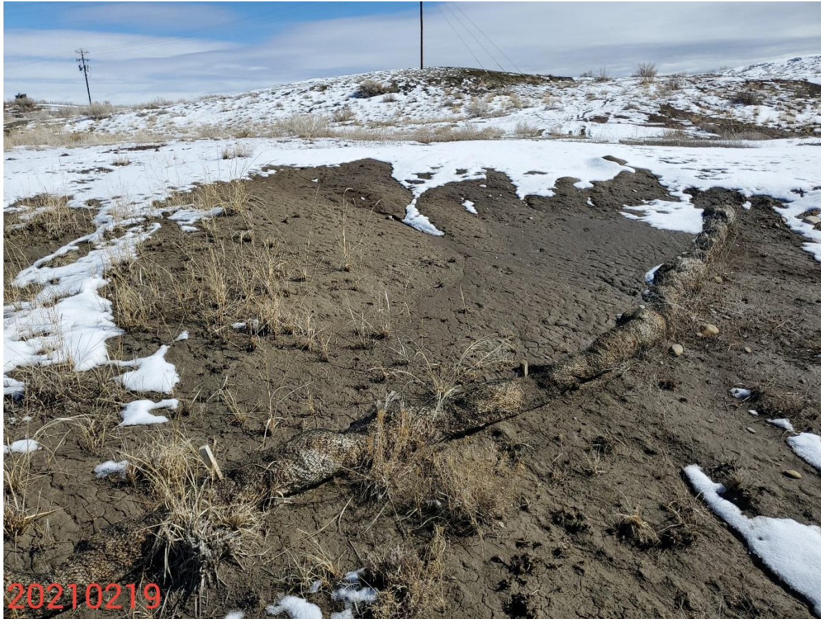
Photo 7: Photo taken from the southern areas of the Location, facing east. Photo shows stormwater and erosion control measures are missing or insufficient to stabilize soils.
