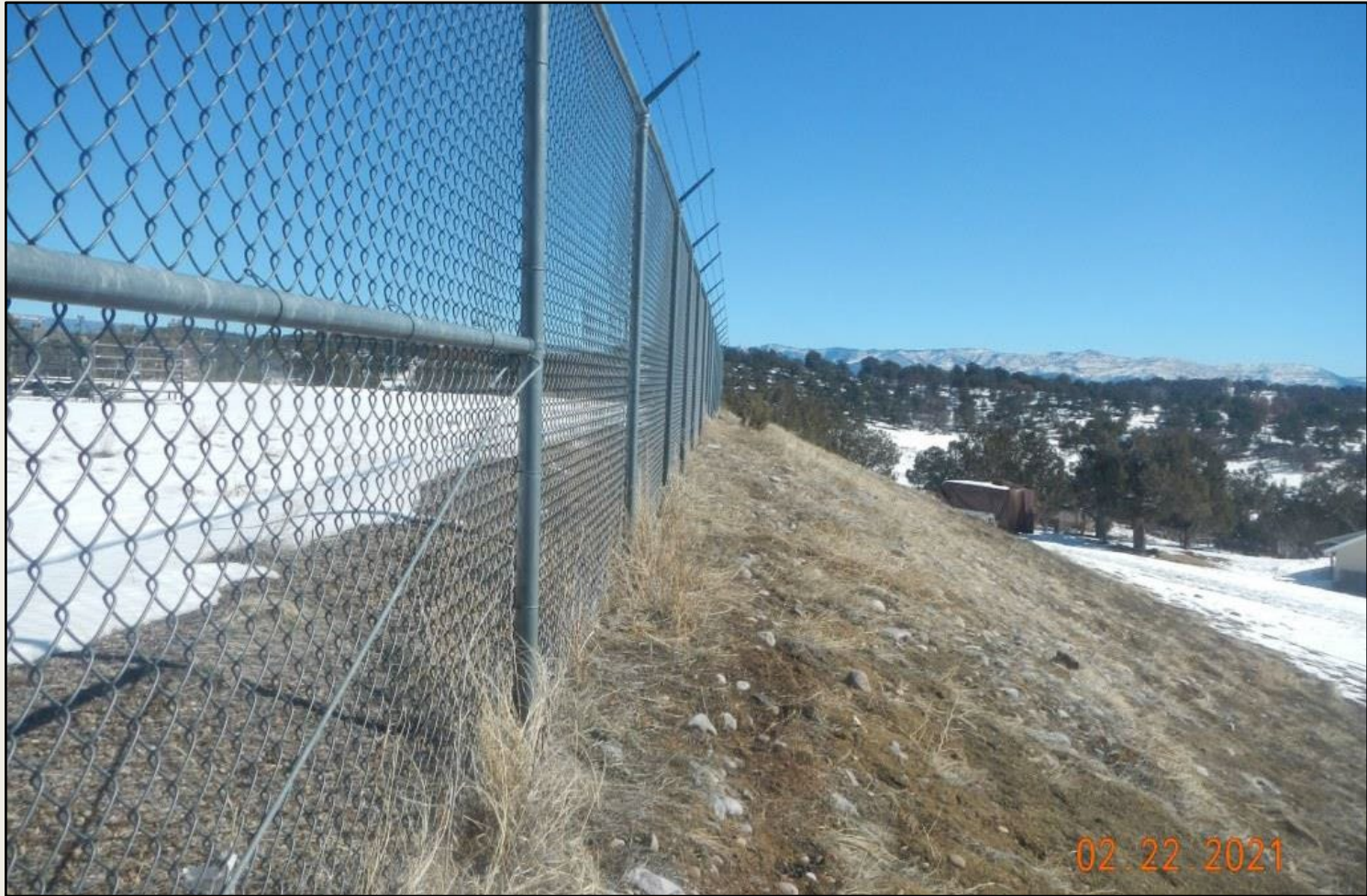
Photo 2. View of the southern fill slope facing eastward. Vegetation is progressing with grasses such as western wheatgrass and sand dropseed, as well as forbs such as Heterotheca villosa .
