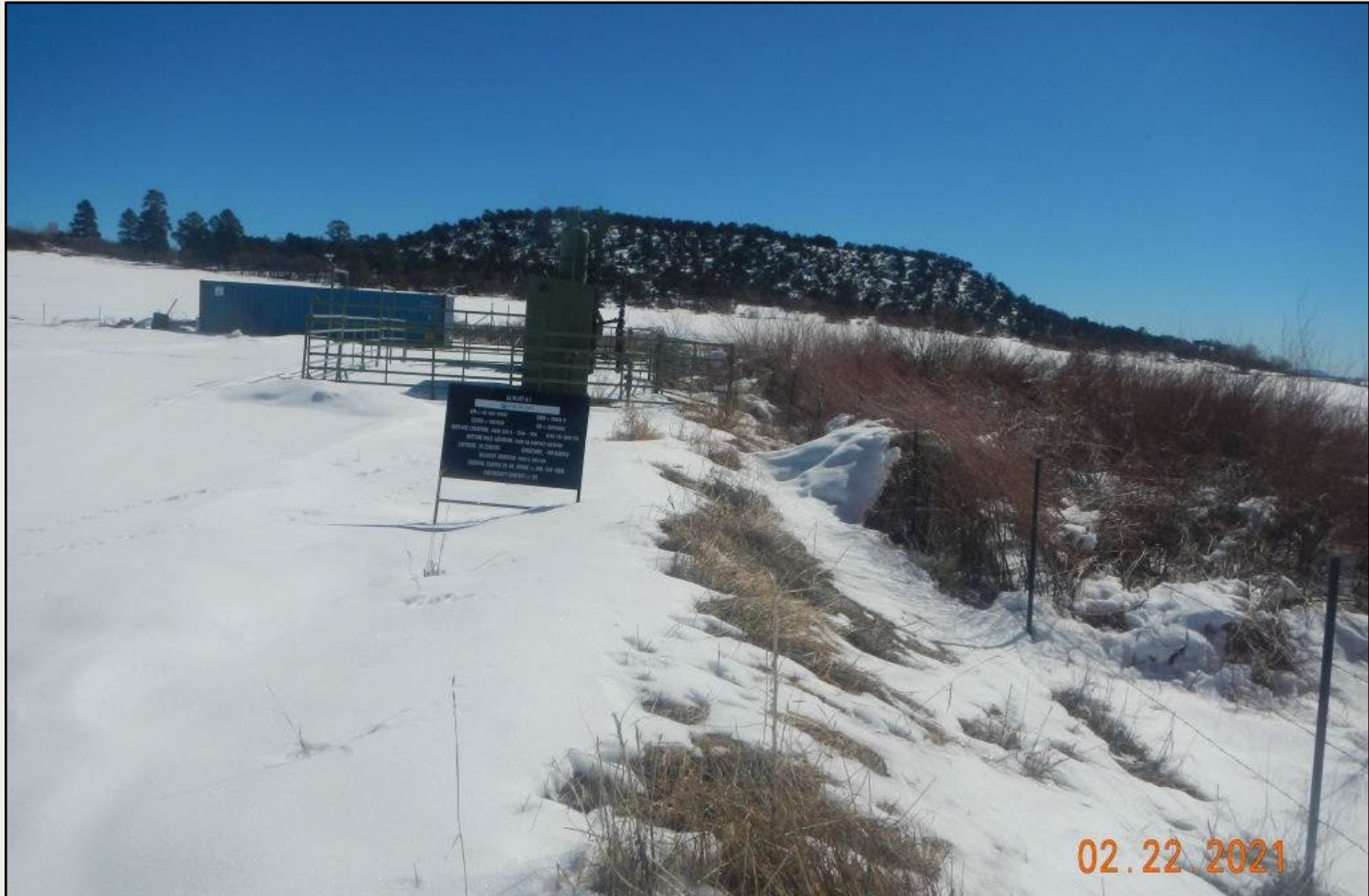
Photo 2. View of the southern fill slope facing eastward. Slope largely snow covered. Perennial vegetation such as western wheatgrass observed in gaps through snow.
