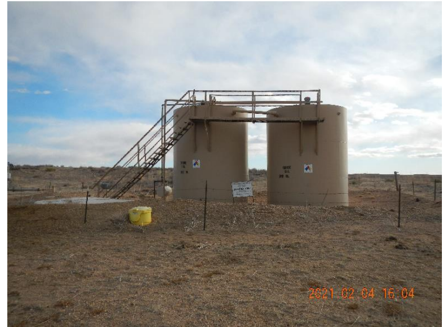
Photo 2: View of tank battery.
