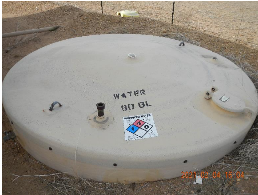
Photo 3: Produced water fiberglass tank.
