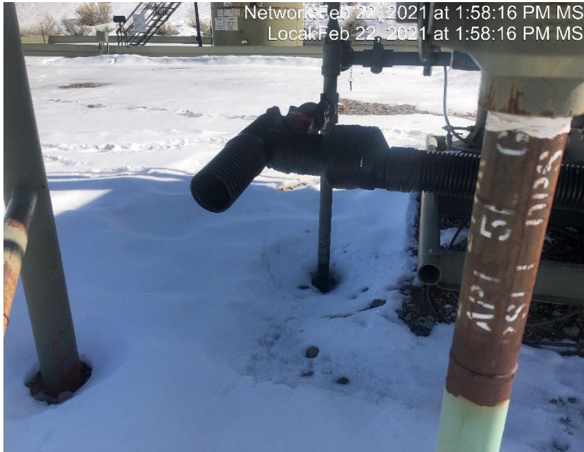
Photo #2950 Flow line heating insulation open ended and not capped.
