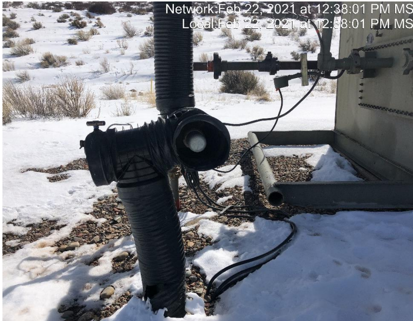
Photo #2944 Multiple flow line heating insulation open ended and not capped.
