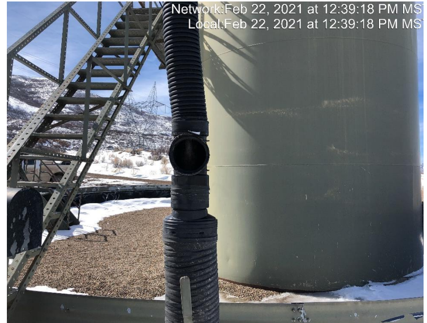
Photo #2945 Multiple flow line heating insulation open ended and not capped.
