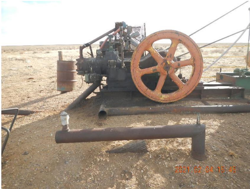
Photo 5: View of gas operated prime mover and supply gas flowline.
