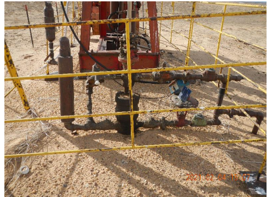
Photo 4: View of wellhead and wellhead tree. Production flowline comes off R side of tree.
