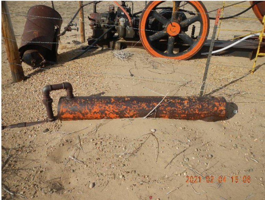
Photo 3: Supply gas dryer vessel with flowline.
