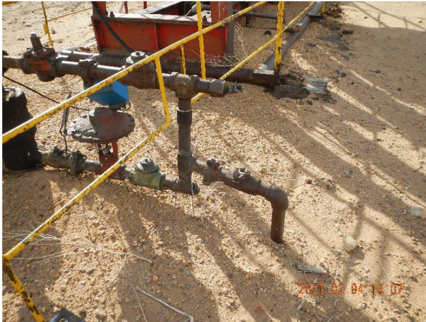
Photo 5: Flowline from wellhead.
