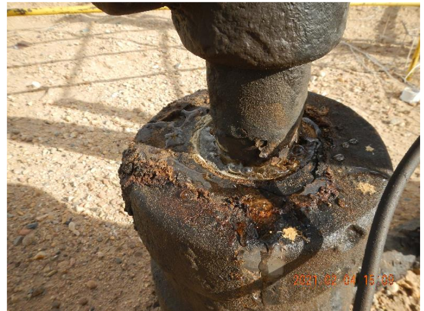
Photo 6: Well venting at cap.
