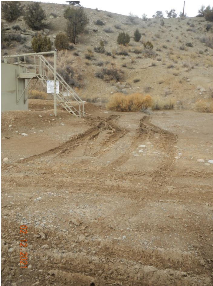
Photo#3: Rutting on portions of site.
