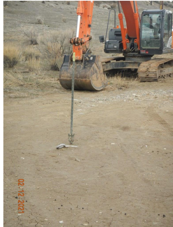
Photo#4: Anchor not marked with bright color.
