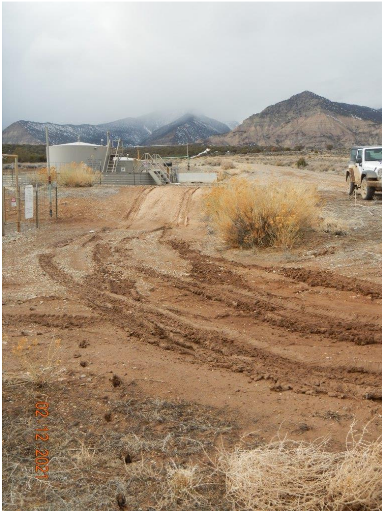
Photo#6: Rutting on equipment area track.
