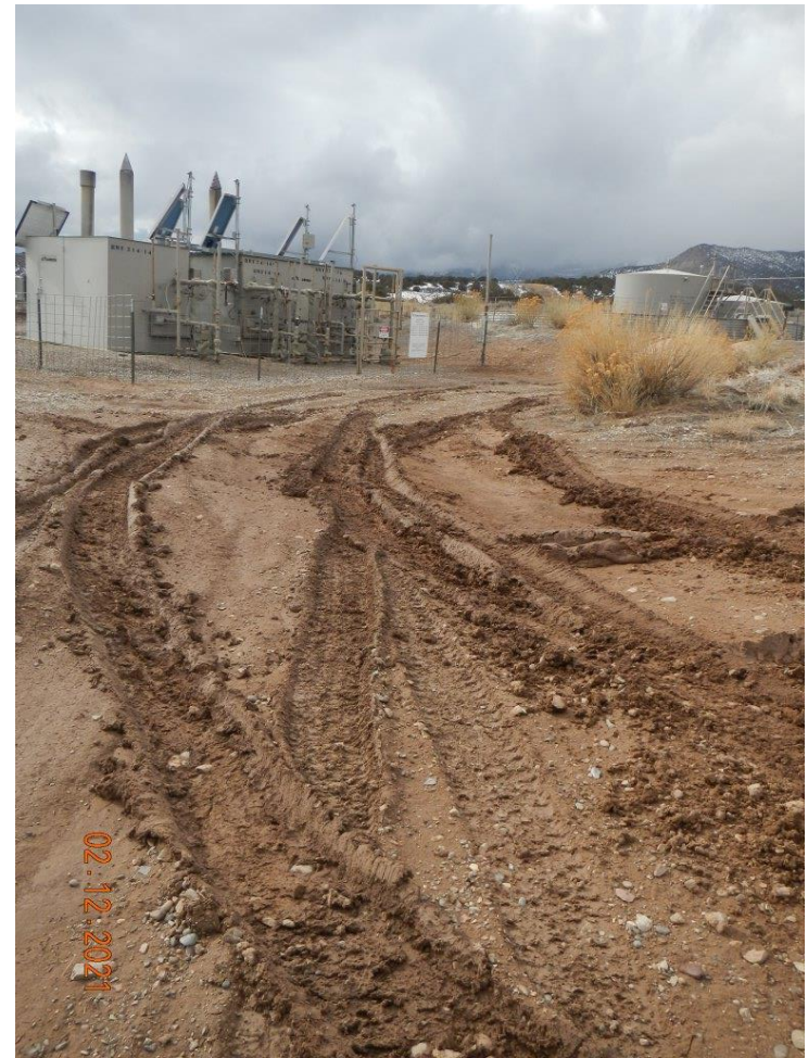
Photo#7: Rutting on equipment area track.
