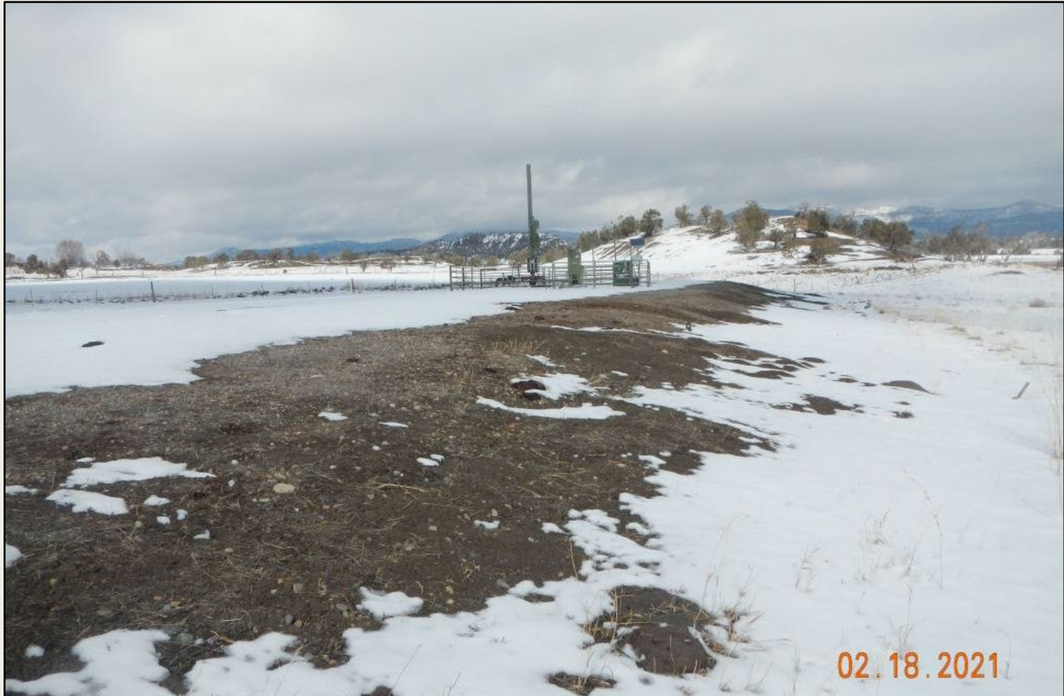
Photo 2. View of the southern fill slope facing eastward. Revegetation is grazed and dormant at this time. However, it is evident that portions of the fill slope are bare. Revegetation needs to be monitored during the active growing season and seeding conducted where vegetation is not becoming established.
