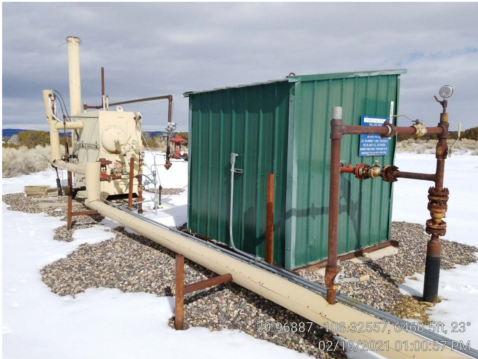
Photo 3. Meter building & separator.
