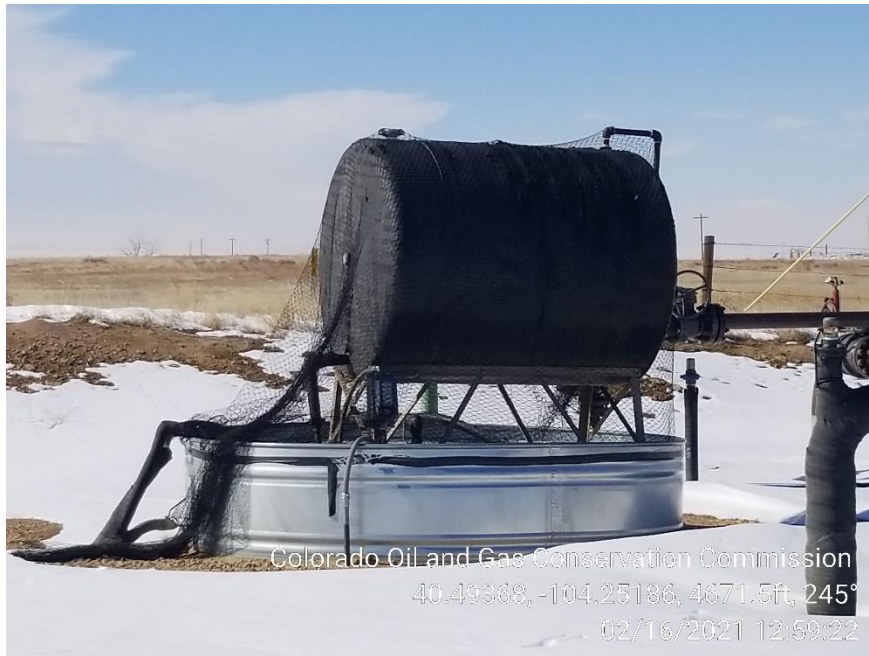
Photo 5 – Wildlife Netting has been installed
