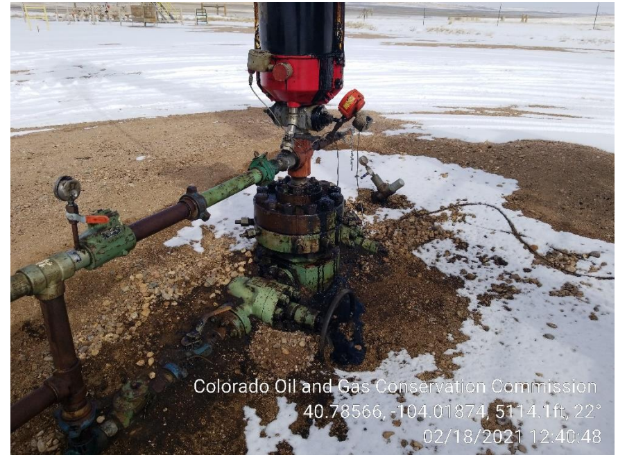
Photo 6 – Stained Soil at Wellhead
