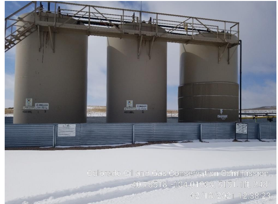
Photo 2 – Tank Battery
