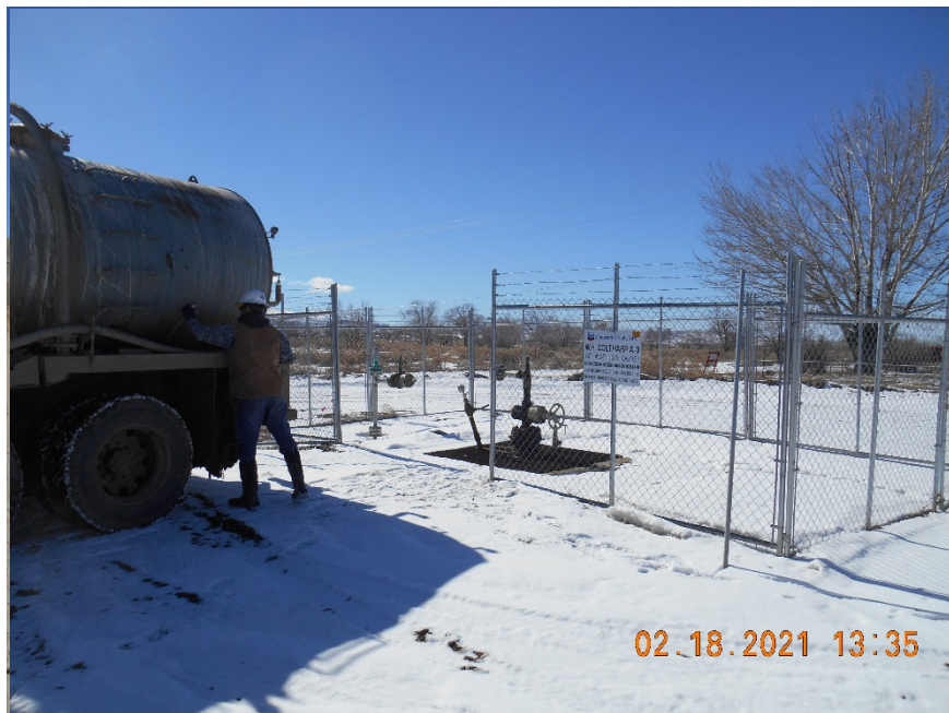
Injection wellhead. Temporarily Abandoned
