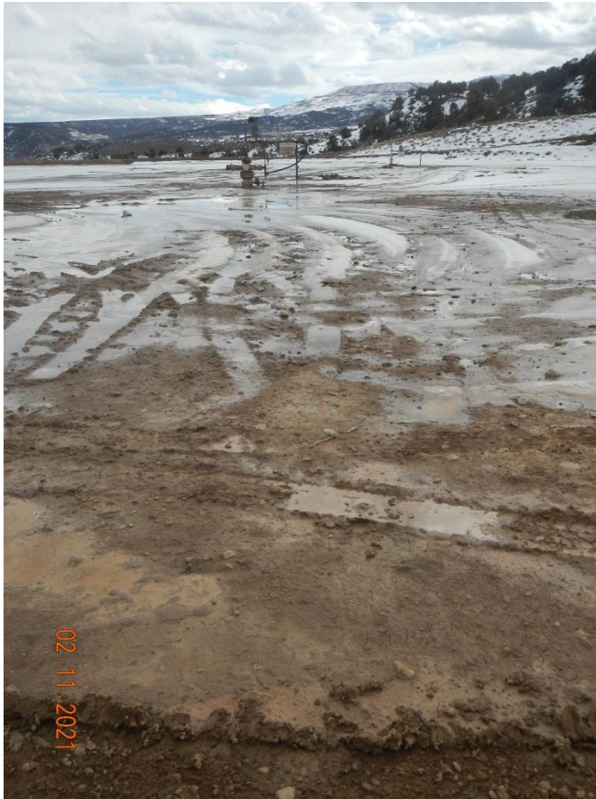
Photo#11: Ponding, rutting on pad.
