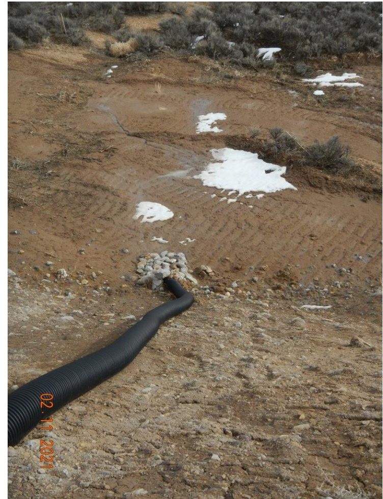
Photo#6: Flexible drain discharges at base of Fill.
