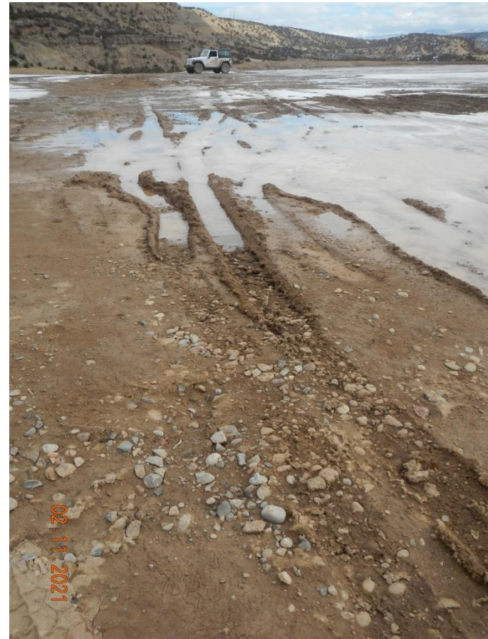
Photo#12: Ponding, rutting on pad..
