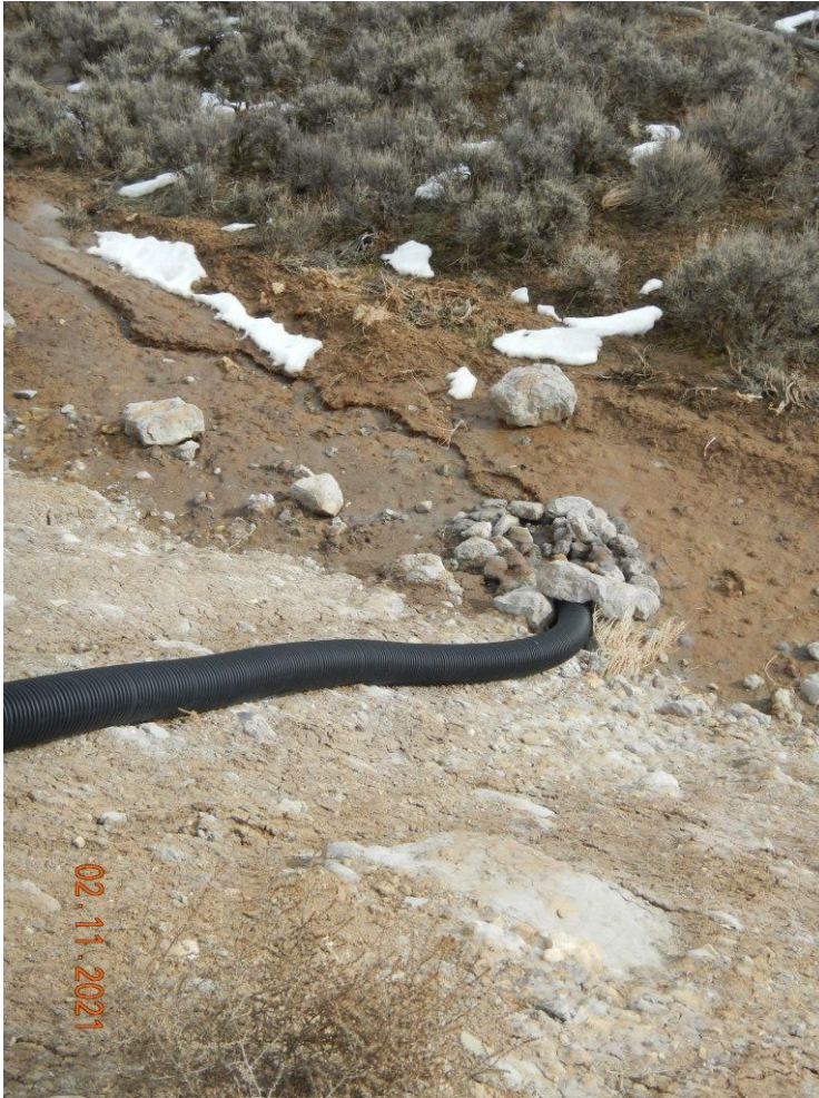
Photo#5: Flexible drain discharges at base of Fill.
