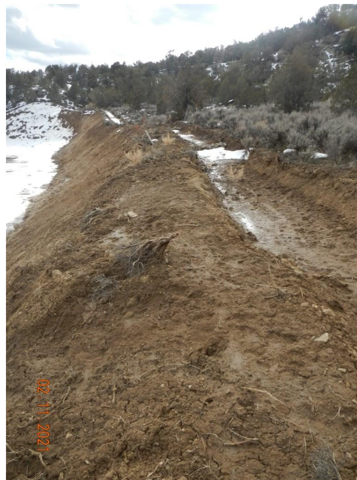
Photo#10: Diversion BMP installed along top of cut .
