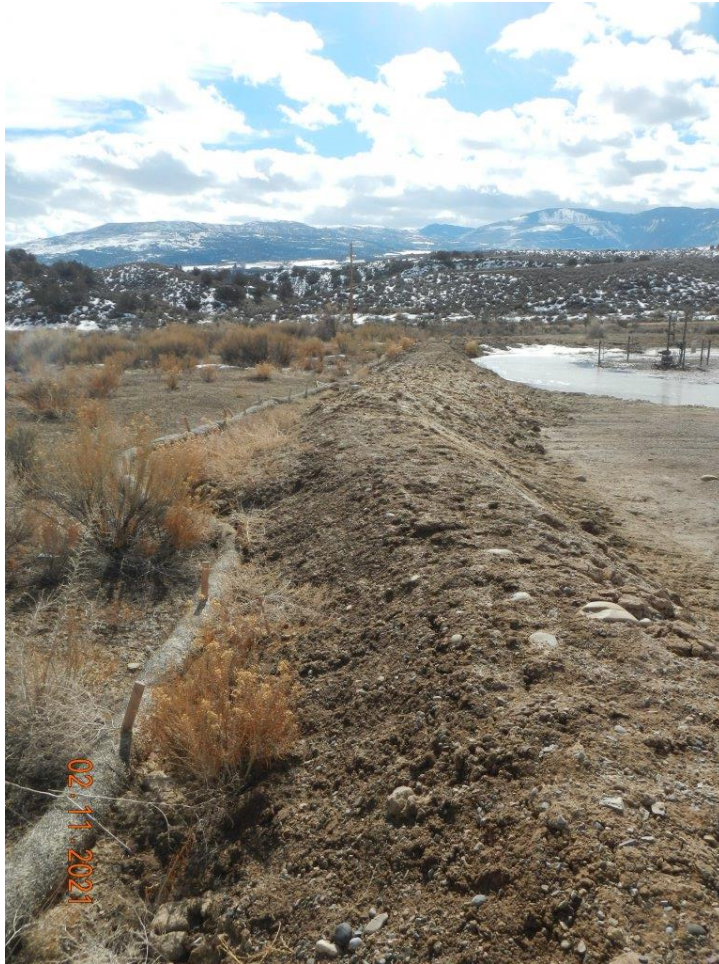
Photo#6: East perimeter berm and wattles.
