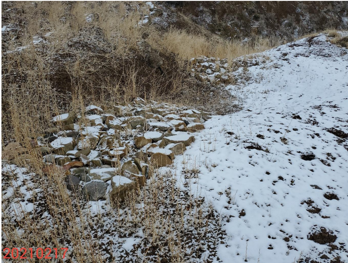
Photo 5: Photo taken from the southeastern interim areas of the Location. Photo shows example of multiple sediment traps installed on the south and eastern ends of the Locaiton.
