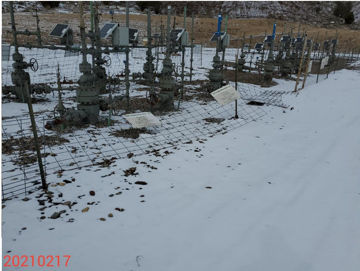
Photo 8: Photo shows fencing panels along wells are in disrepair.
