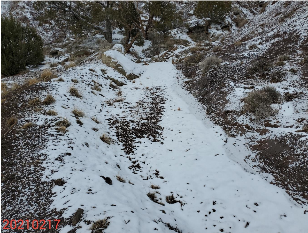
Photo 6: Photo shows perimeter stormwater ditch and berm to manage stormwater runoff.
