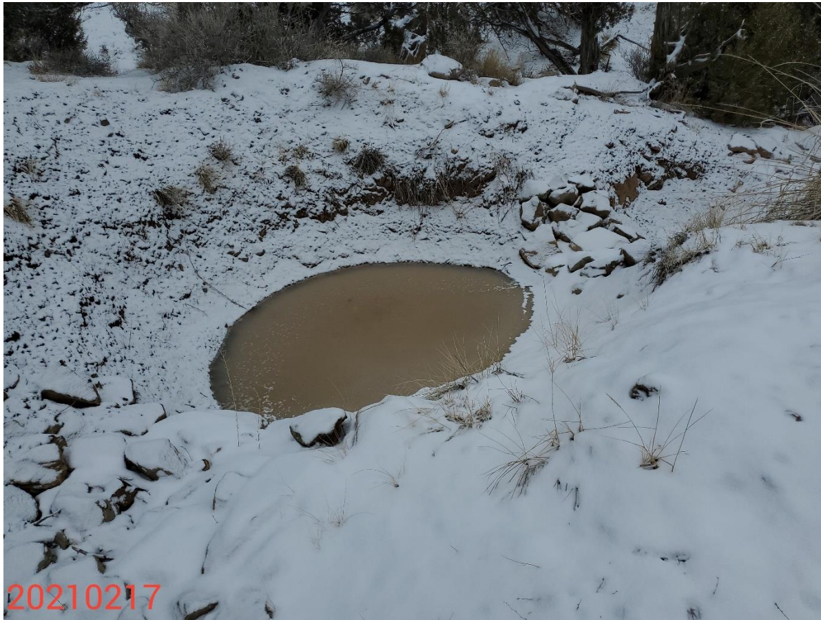
Photo 4: Photo shows sediment trap observed on the east end of the Location.
