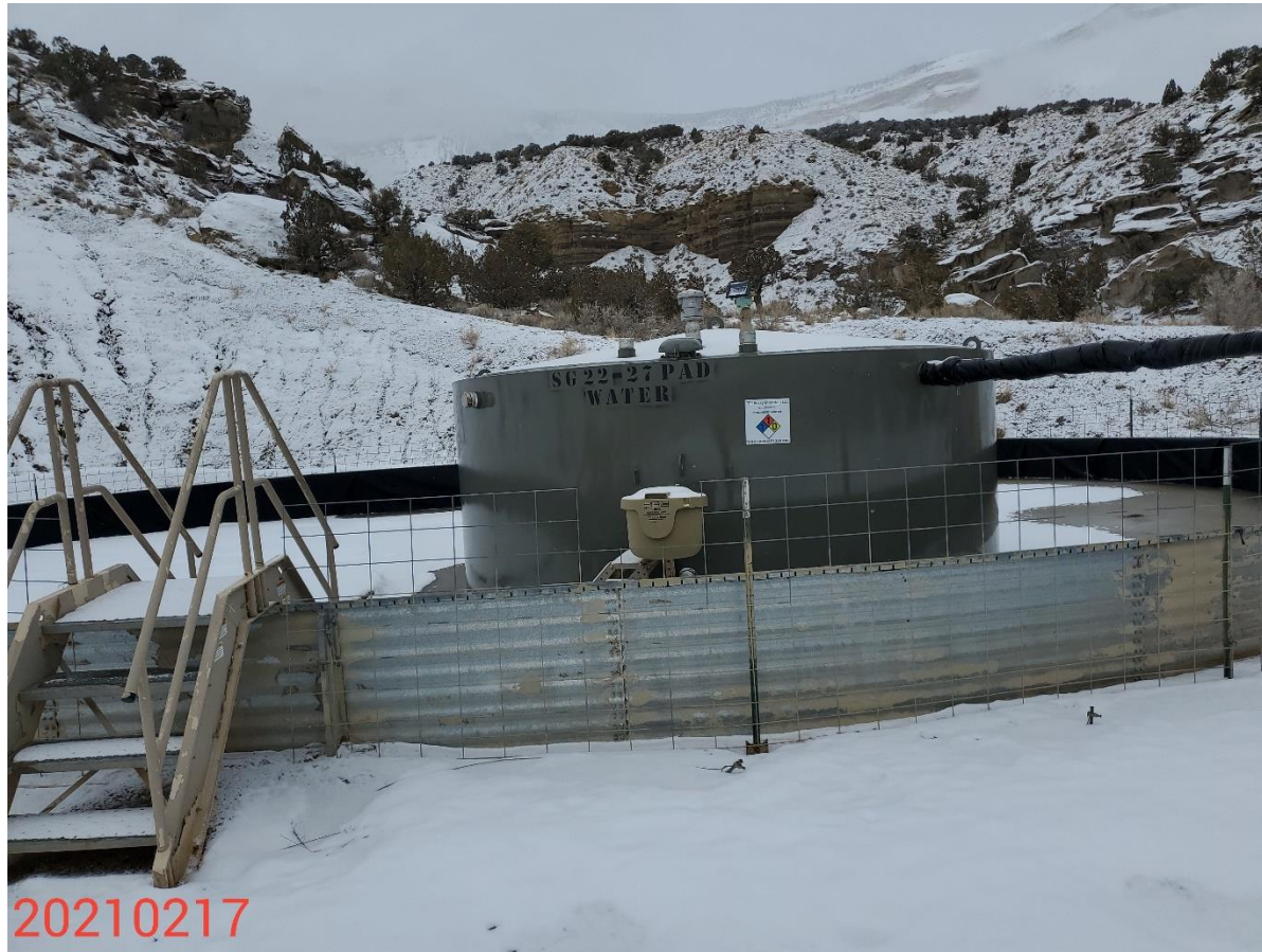
Photo 5: 200 bbl produced water tank and containment bmp.
