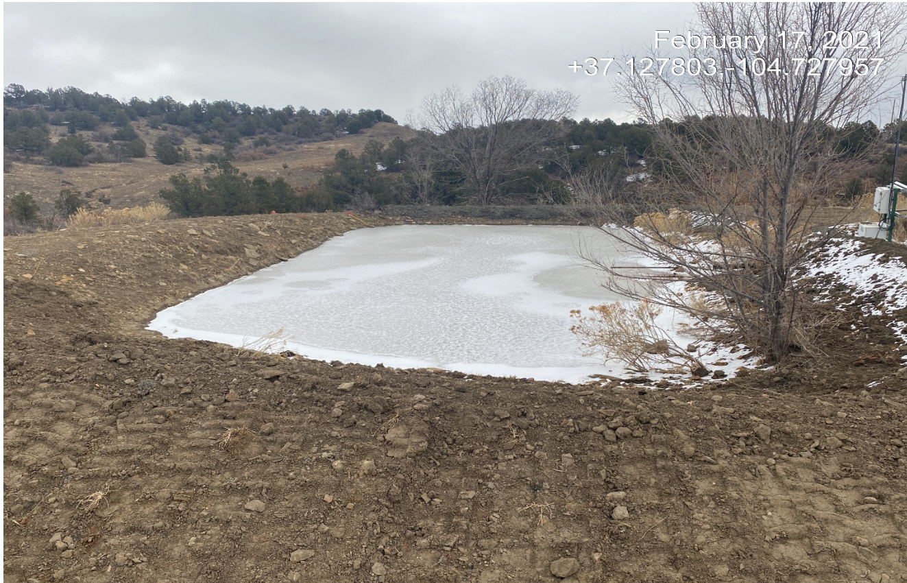
Photo 3. Facing toward the pit. Water level was about 6inches from the freeboard marker.
