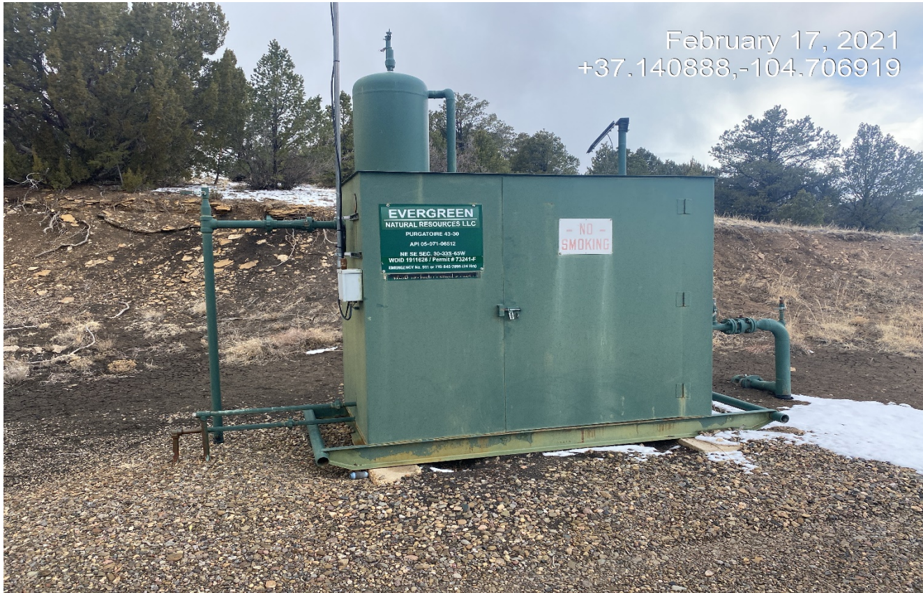
Photo 3. Well sign posted at meter shed.
