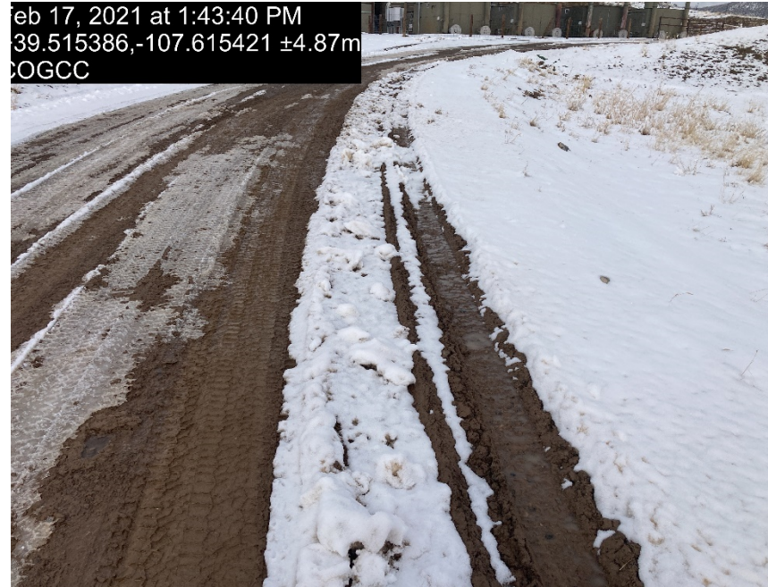
Lack of stabilization/entrance looking north into location
