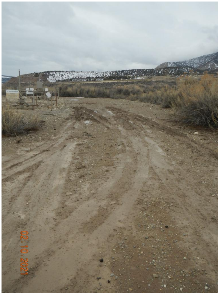
Photo#2: Rutting, sloppy conditions at Well head area.
