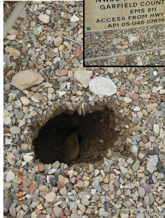
Photo#5: Developing subsidence/ tunneling.
