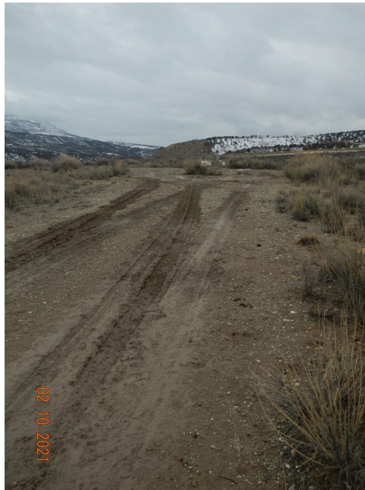
Photo#3: Rutting, sloppy conditions leading into Well head area.
