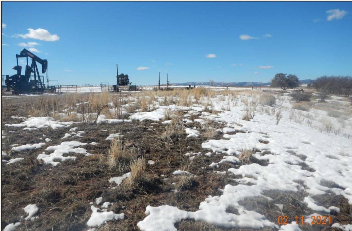
Photo 2. View of the northern fill slope from the northeastern corner facing westward. Revegetation appears to be progressing with crested wheatgrass observable.
