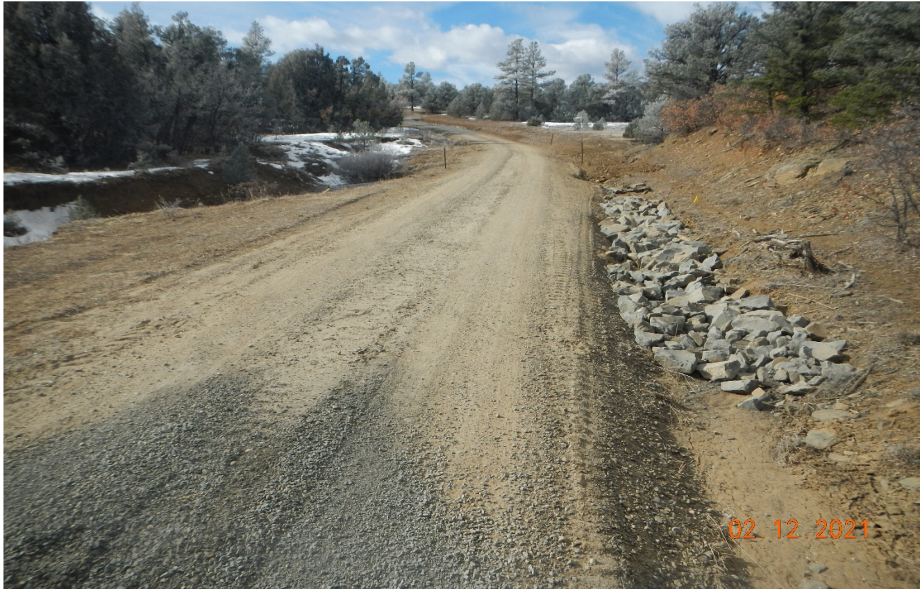
Photo 3. Facing west along the main road. The side of the road has been repaired with BMP's installed.
