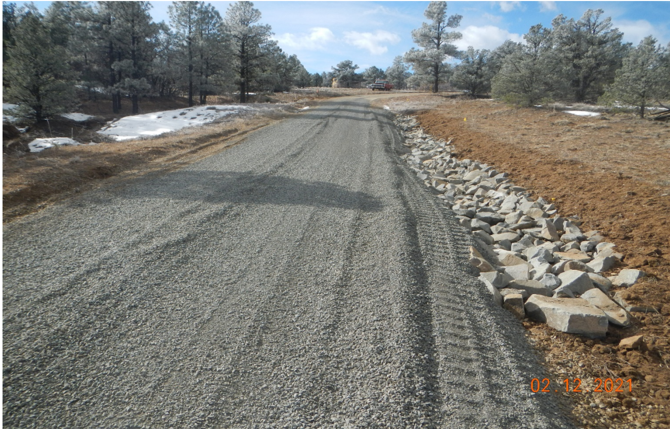
Photo 4. Facing southwest along the main road. Gravel has been installed along this area of the road. Rock rip/rap has been installed for erosion control.
