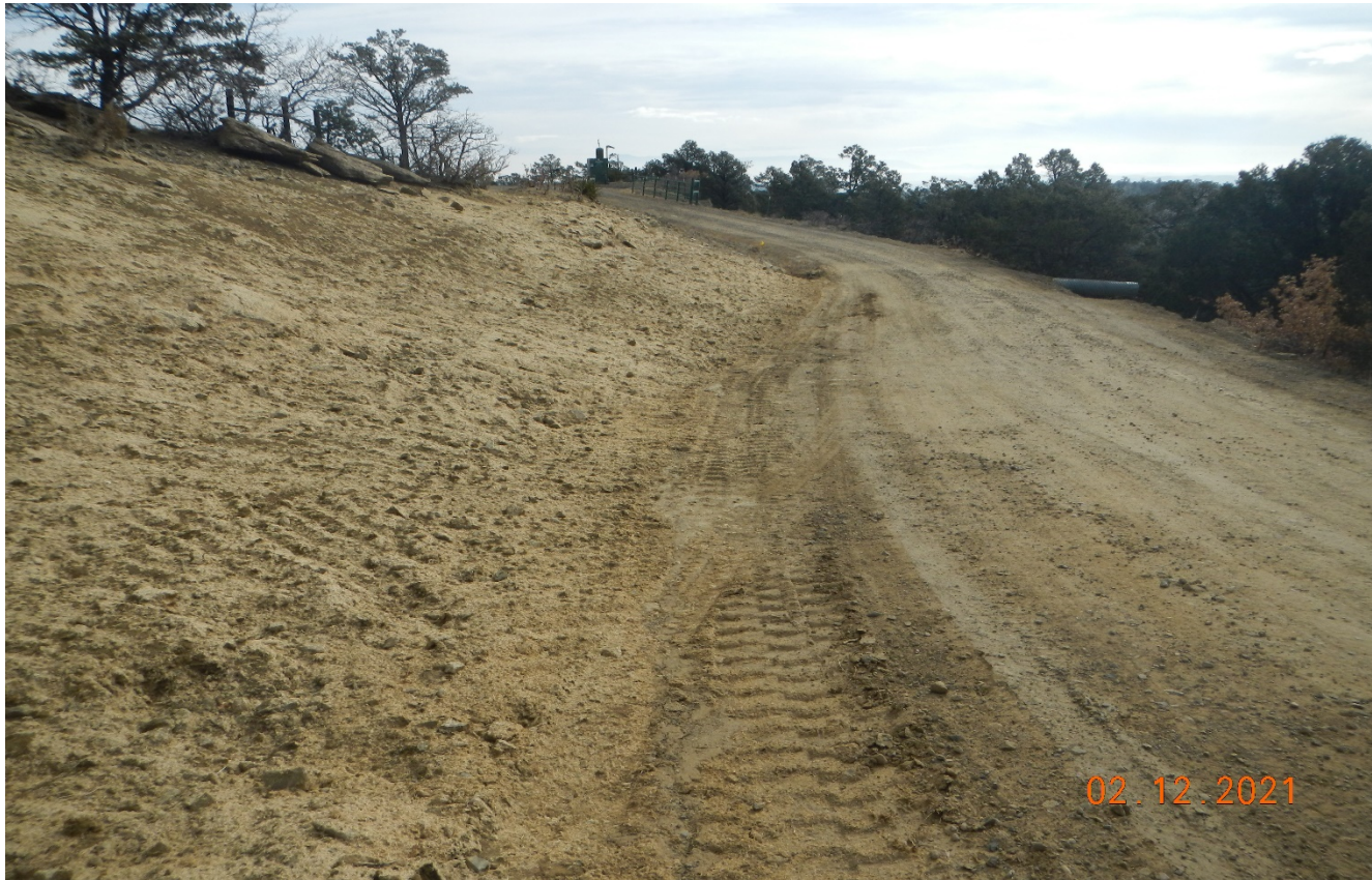
Photo 6. The side of the access road has been seeded and hydromulched.
