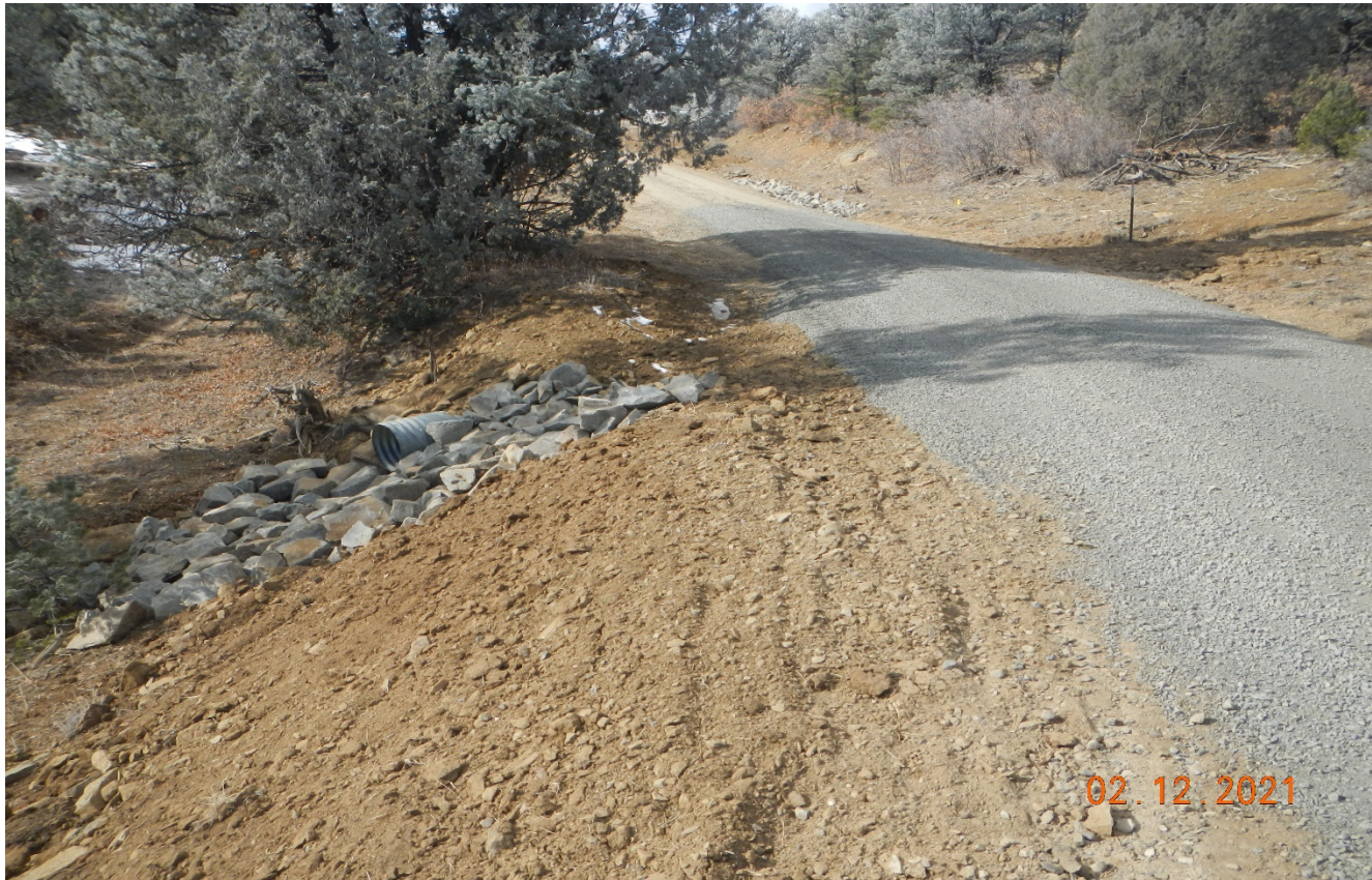
Photo 2. Outlet protection has been installed at Lat/Long:37.15900,-104.81291.
