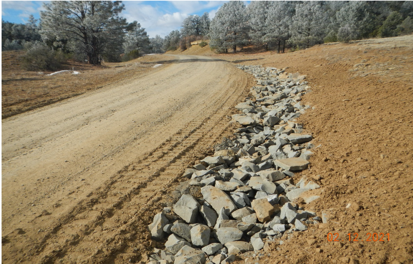
Photo 1. Facing west along the main road. Erosionalong the road has been repaired and BMP's have been installed and maintained.
