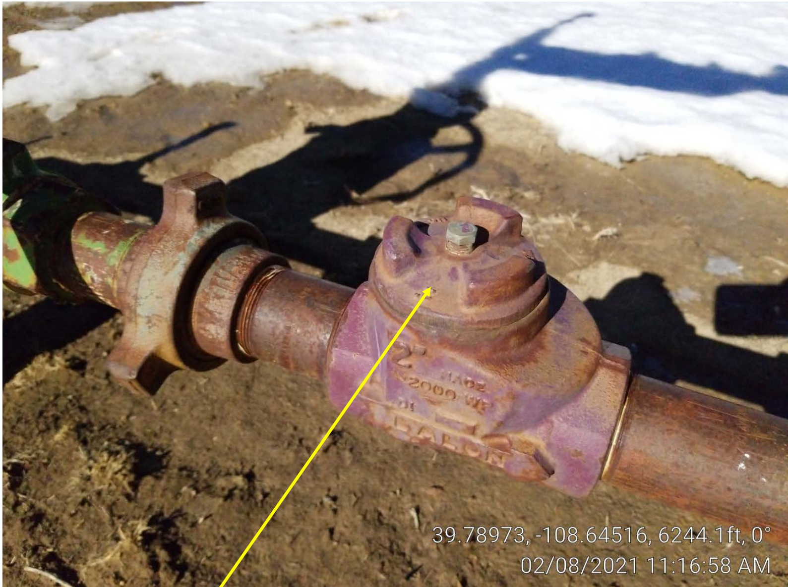
Photo 2. Gas leak.
