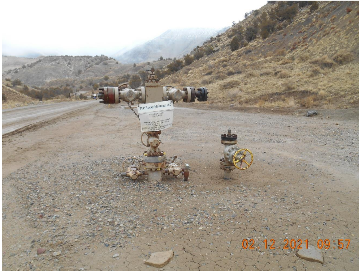
Injection wellhead. Temporarily abandoned.
