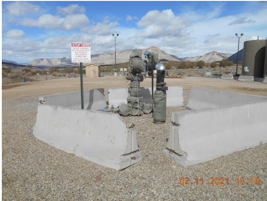
Injection wellhead with cement barricades
