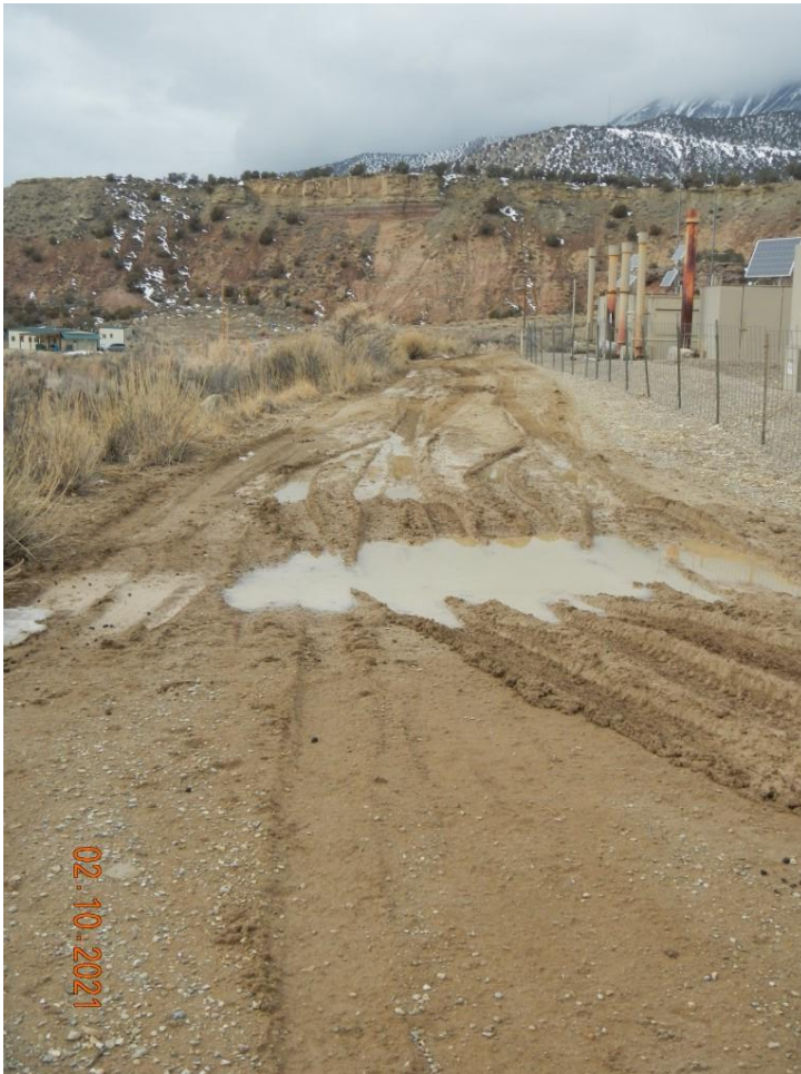
Photo#2: Rutting, degradation of pad surface.
