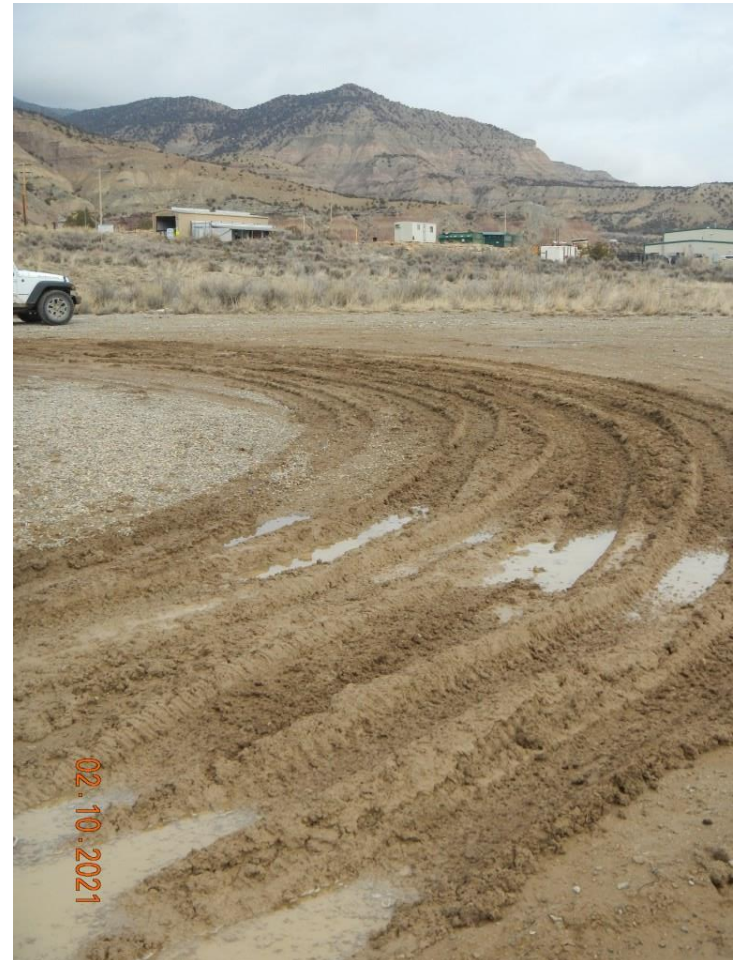
Photo#3: Rutting, degradation of pad surface.
