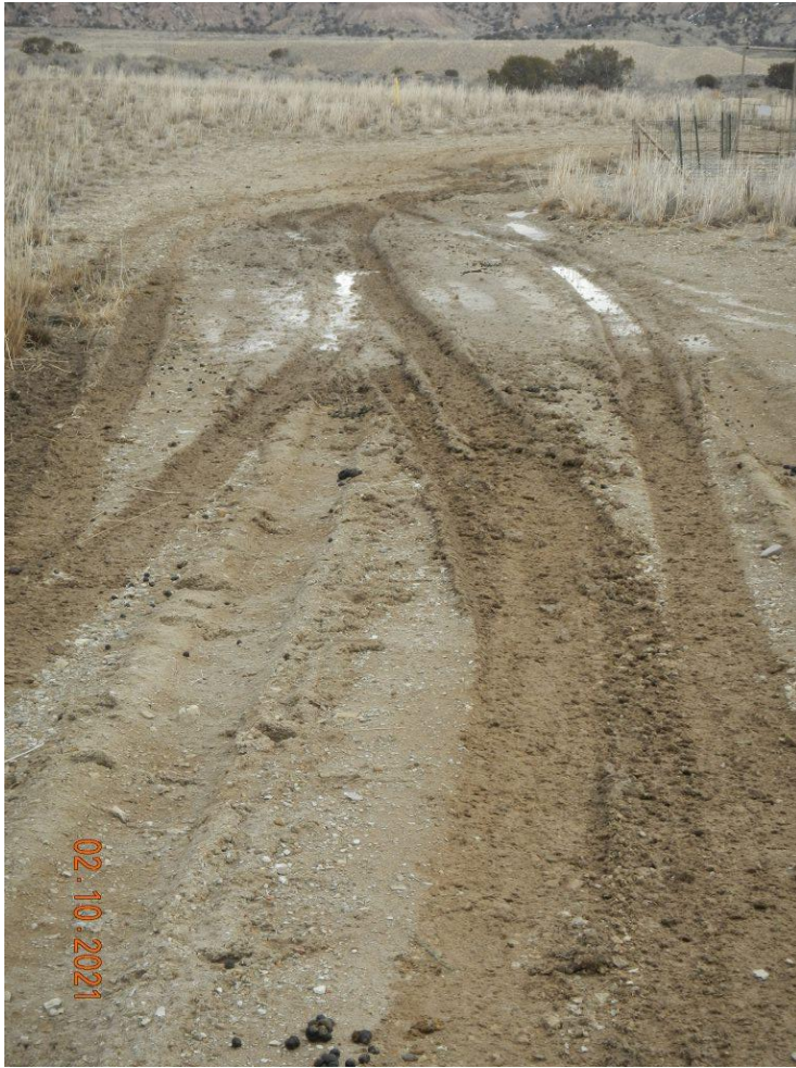
Photo#2: Rutting, degradation of pad surface.
