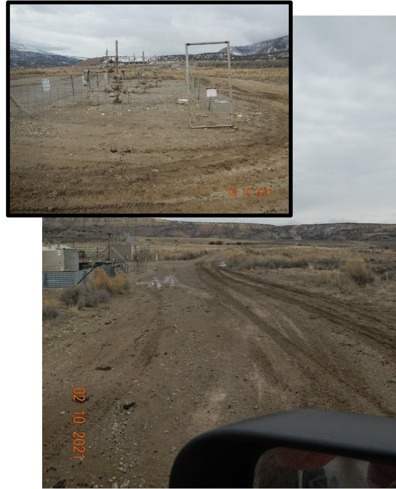
Photo#3: Rutting, degradation of pad surface.
