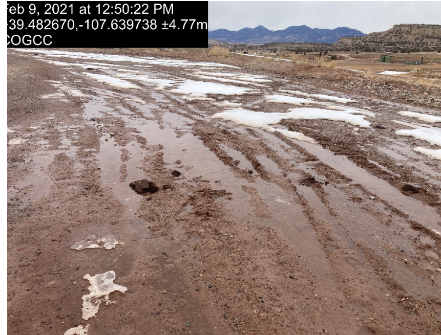
Lack of stabilization from follow up inspection
