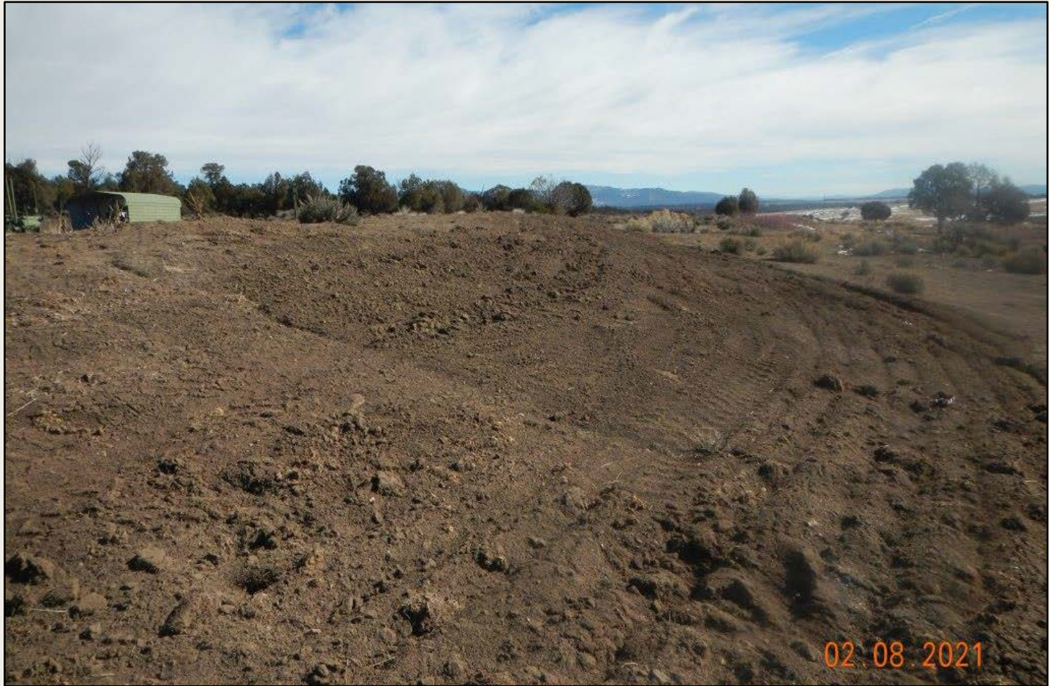
Photo 2. View of the southern fill slope from the southwestern corner facing eastward. Revegetation is conducted. Slopes are tracked. Mulching is not present. Revegetation needs to be monitored. Cattle exclusion is recommended.
